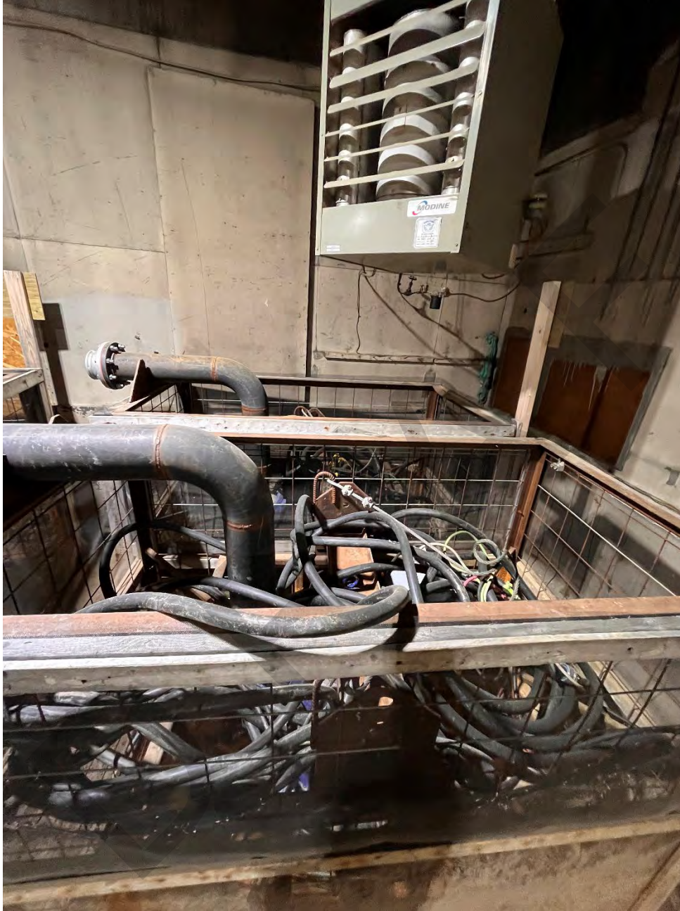
Figure 4: Wiring for each pump is contained in the fish screen.
