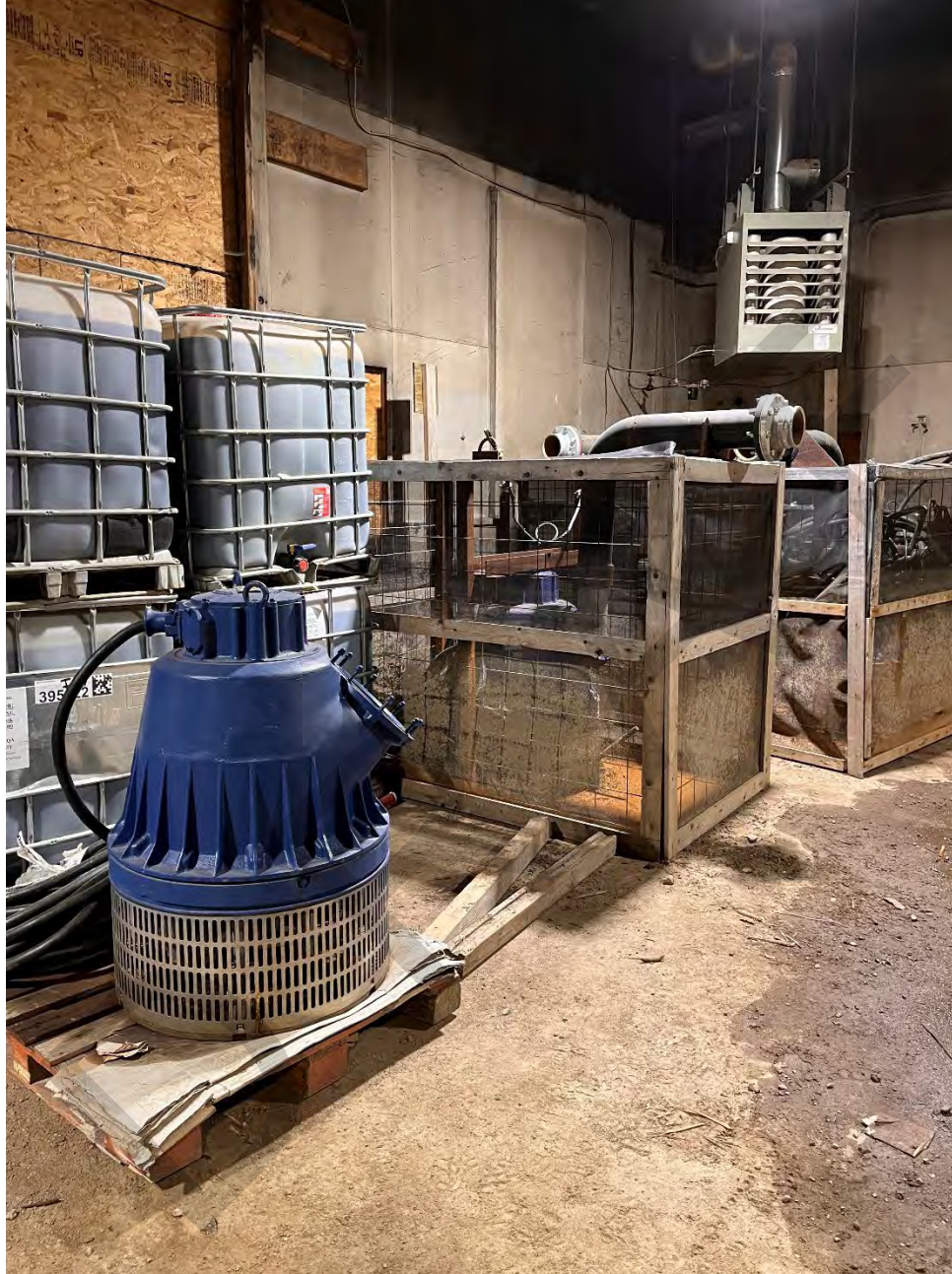
Figure 1: 3 pumps in fish screens. Pump not in fish screen is the backup 4th pump. At Apex Warehouse.
