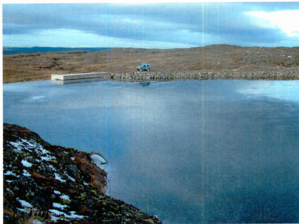
Photograph No. 4 – Lake Geraldine Reservoir, looking northwest to embankment portion of dam. Spillway section is at extreme left.
