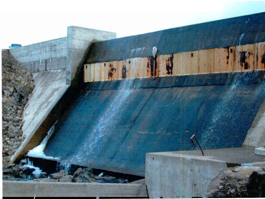
Photograph No. 7 – Overview of north end of Gravity elevation and Spillway elevation. Note leaching cracks on Gravity face.
