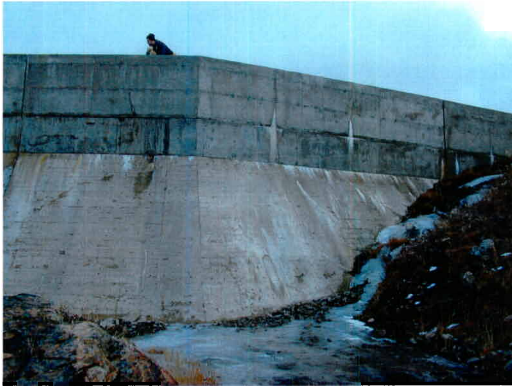
Photograph No. 9 – Overview of south Gravity elevation. Note leaching cracks.
