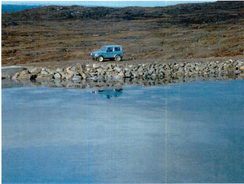
Photograph No. 5 – Close-up of embankment portion at tie-in with Gravity section (at left), upstream face.
