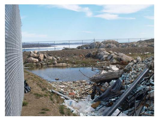
On site runoff detention pond on northeast side of landfill site. Runoff is naturally flows from this pond to runoff detention pond at south west corner.
