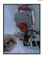
STEP 3. Use a magnet to determine if it is indeed a mercury probe (non-magnetic probes are non-mercury).
