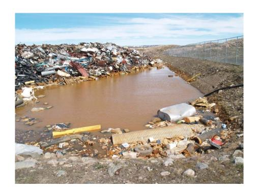
On site runoff detention pond at south west corner of landfill site. Runoff is pumped from this pond to runoff retention pond.
