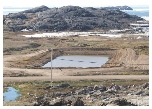
Runoff **retention** pond , south of landfill site, receives runoff from landfill detention pond . Retention pond is sample and discharge twice each year.
