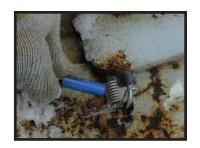
**STEP 5.**Cut or remove any attached wires.
