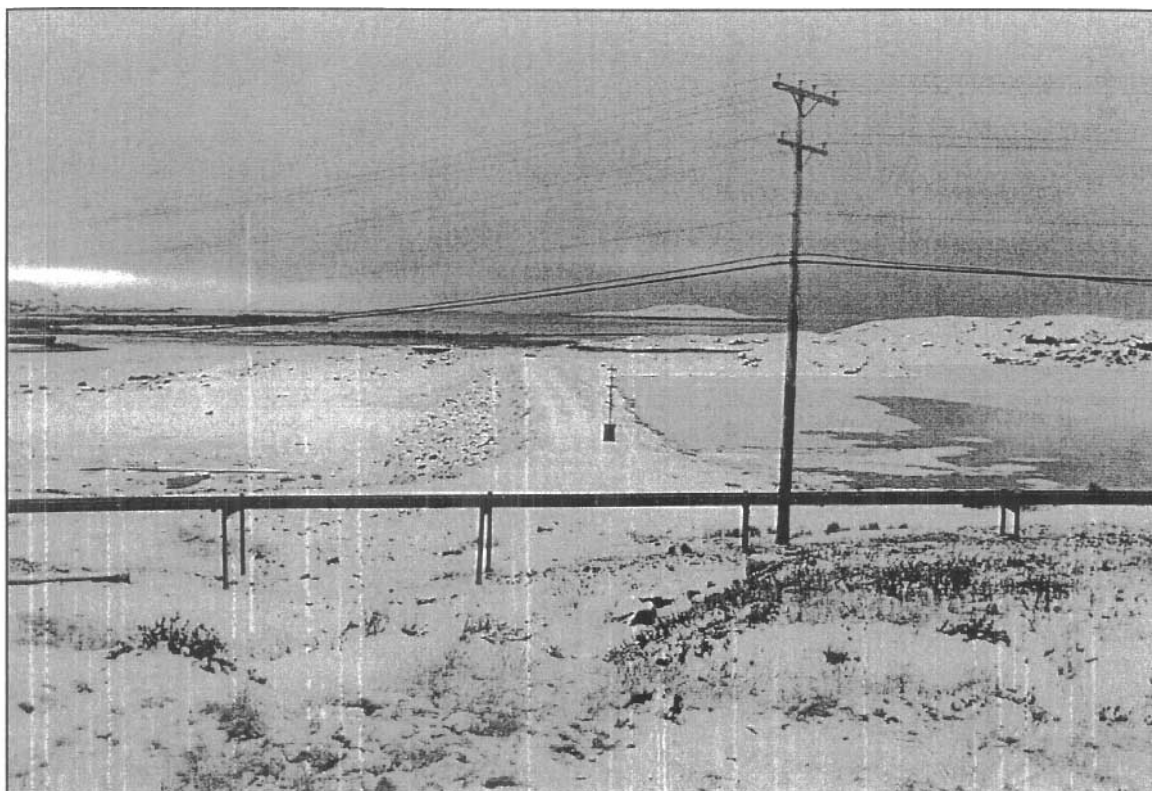
Photo 3 - Looking at The East Dyke of the Sewage Lagoon
