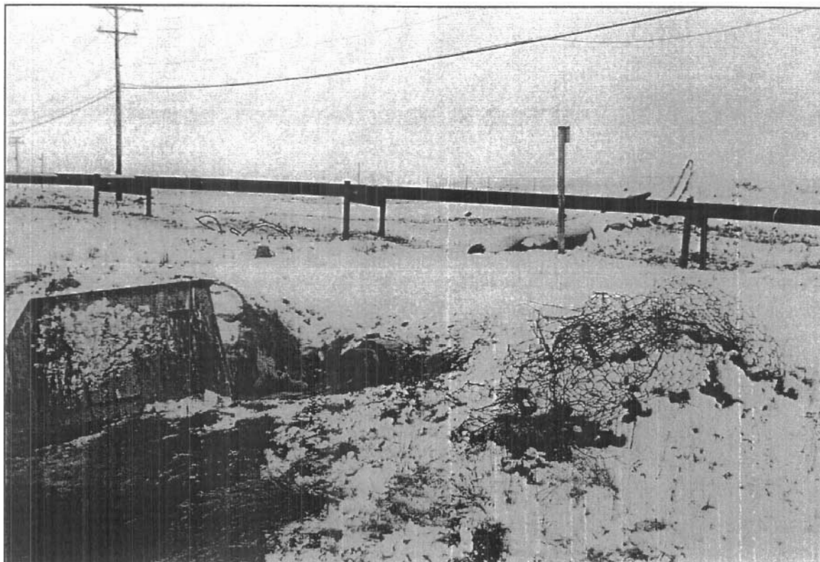
Photo 5 - Discharge Pipe in the Sewage Lagoon (South Side of Lagoon)
