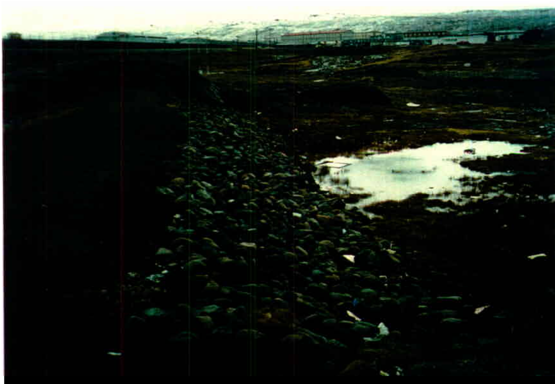
Photo 10 View looking northeast at downstream slope of Southeast Dyke. Some seepage ponding is evident along the toe.
