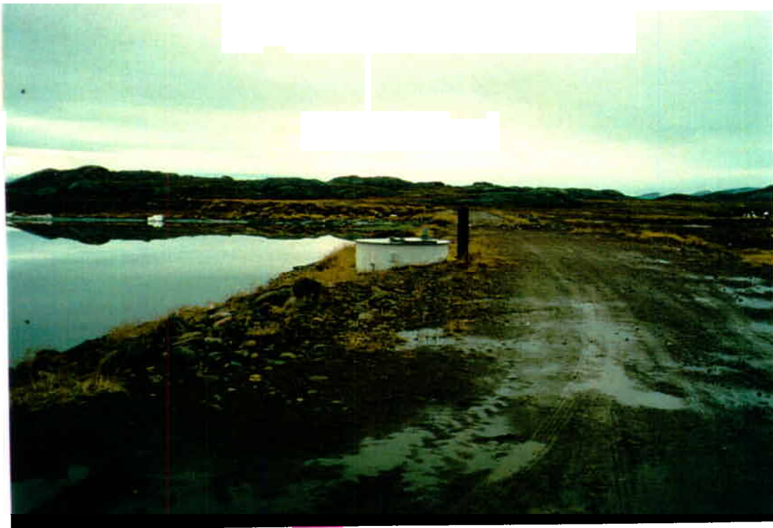
Photo 2 View taken from north end of West Dyke looking south along upstream face and crest of West Dyke. The Discharge Control Structure for the lagoon is in the foreground
