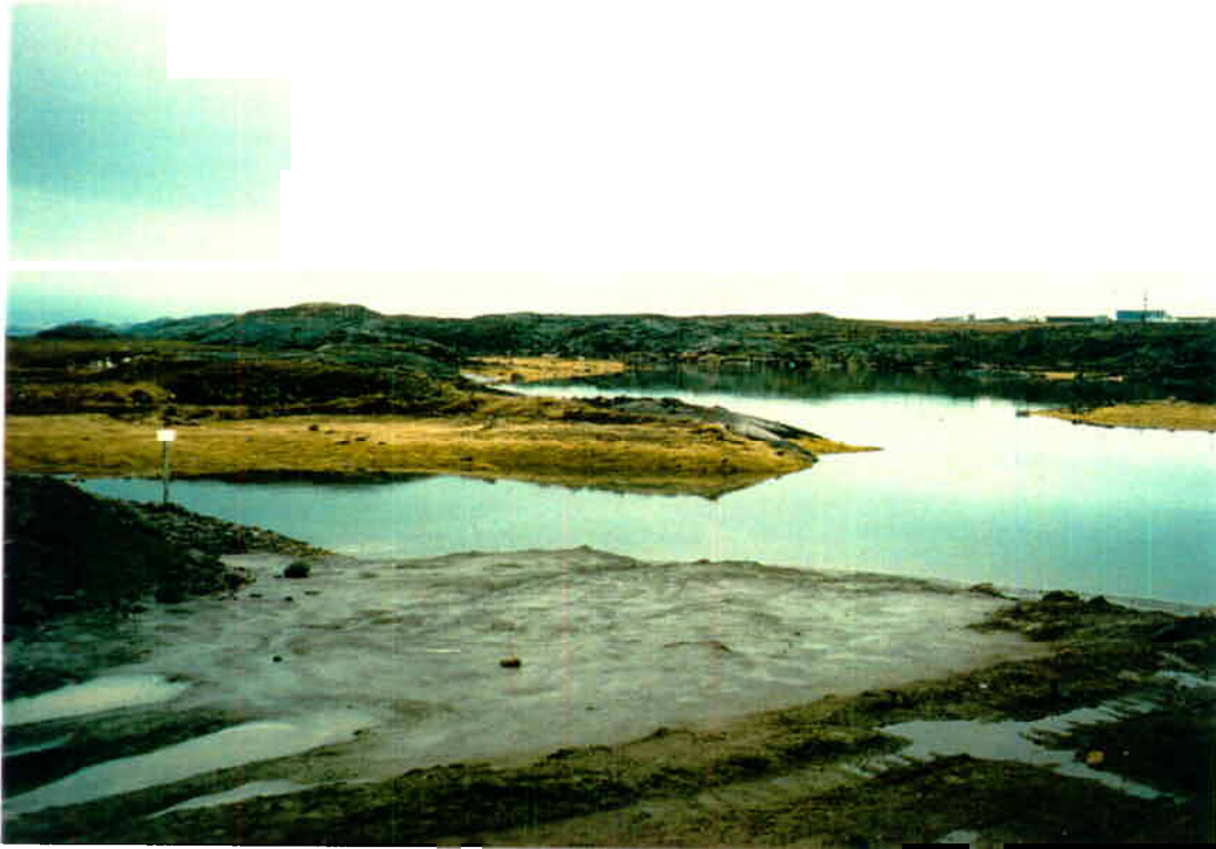
Photo 5 View taken from north end of West Dyke showing area that appears to have been previously breached and was infilled with local silty sand & gravel fill. The fill material appears to be saturated.
