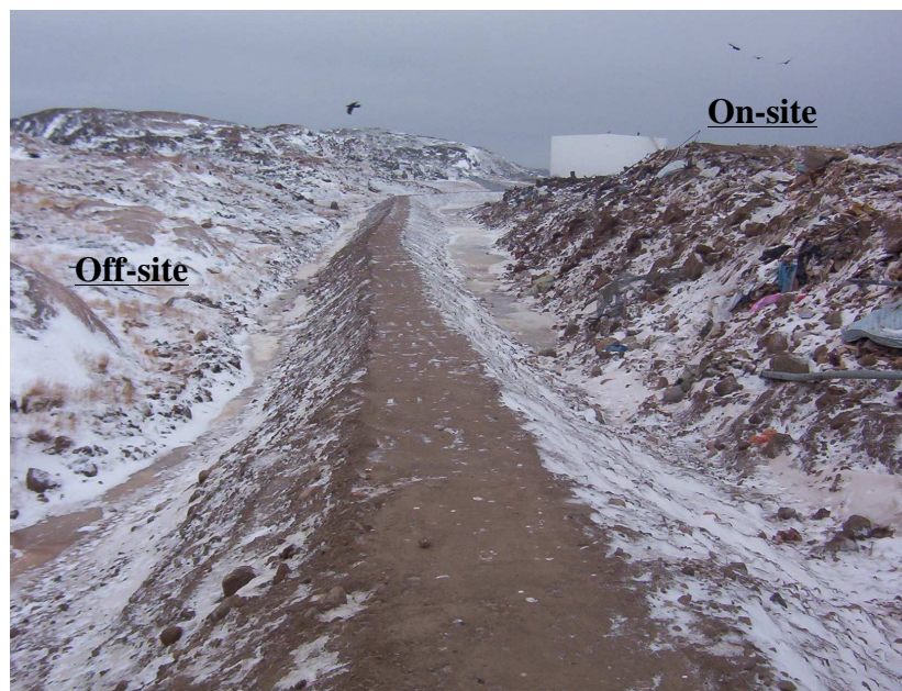
Figure 2-1. Continuous ditches formed with a perimeter berm structure to control on-site and off-site surface runoff at the West 40 landfill site in Iqaluit.
