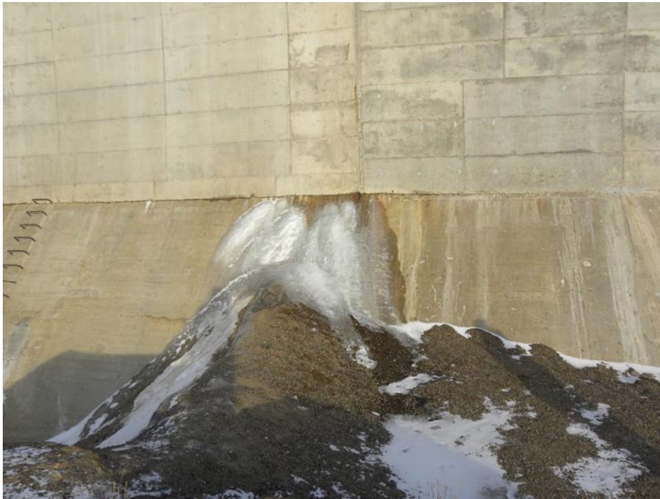
Photograph 5 New leak South of spillway section.
