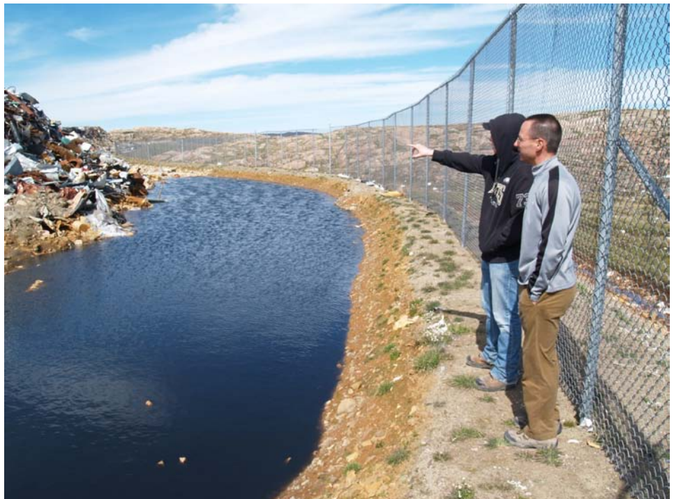
On site runoff detention pond at south east corner of landfill site. Runoff drains from this pond to runoff detention pond at south west corner.
