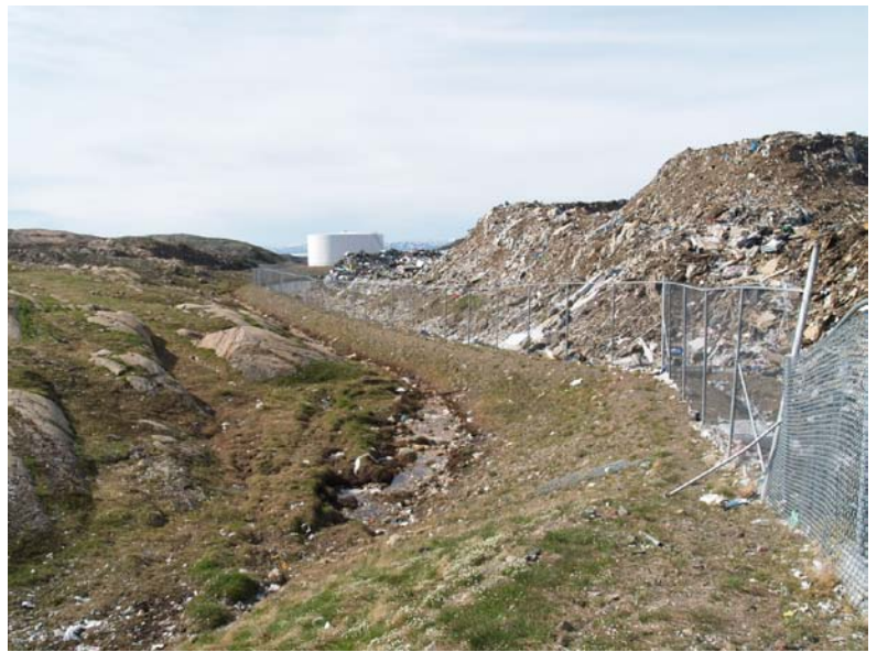
Off site runoff management control system on southeast side of the landfill site (view to south)
