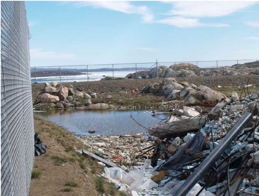
On site runoff detention pond on northeast side of landfill site. Runoff is pumped from this pond to runoff detention pond at south west corner.
