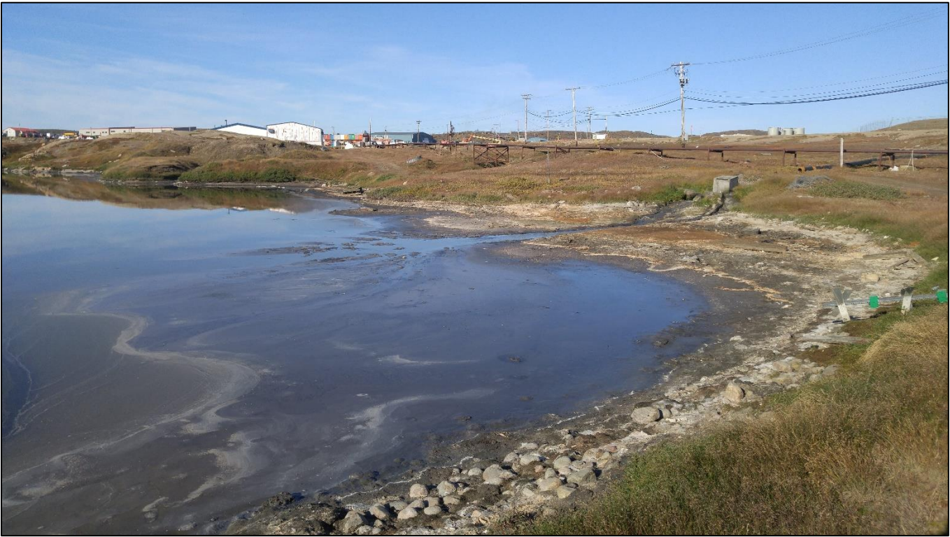
Figure 12 The north east corner of the Iqaluit Lagoon at the influent location was full of sludge. A portion of this area was not accessible by boat due to the extremely shallow beach that has formed. This influent area was in constant operation during the survey.
