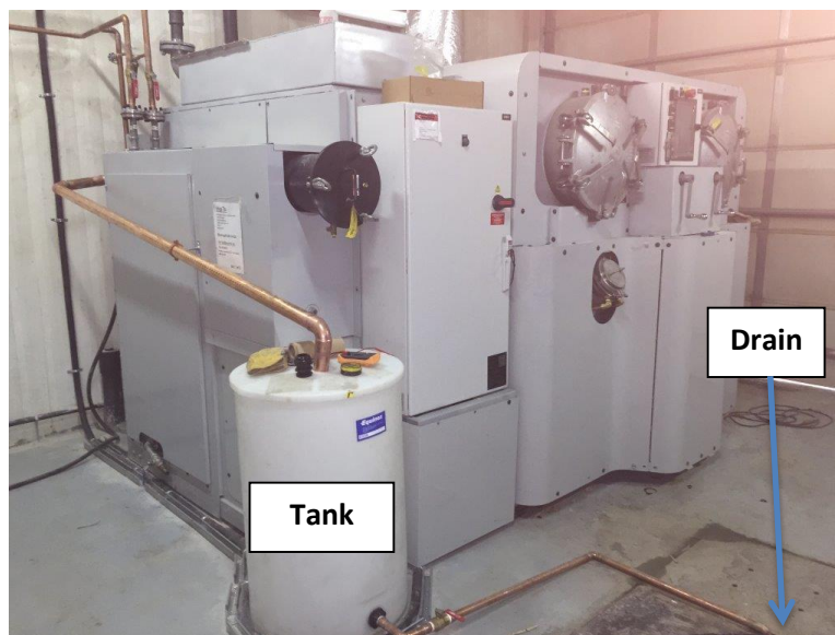
Figure 6: Scrubber drain set-up
