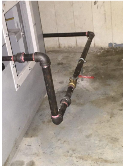
Figure 5: Gravity fed diesel line
