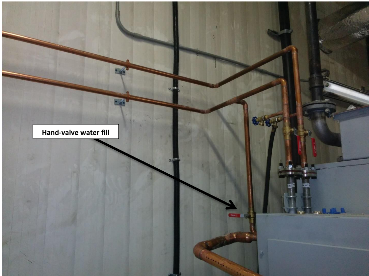
Figure 12: Hand-valve water fill
