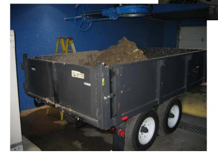
Sewage sludge transportation trailer positioned below discharge channel – note access door at front of trailer.
