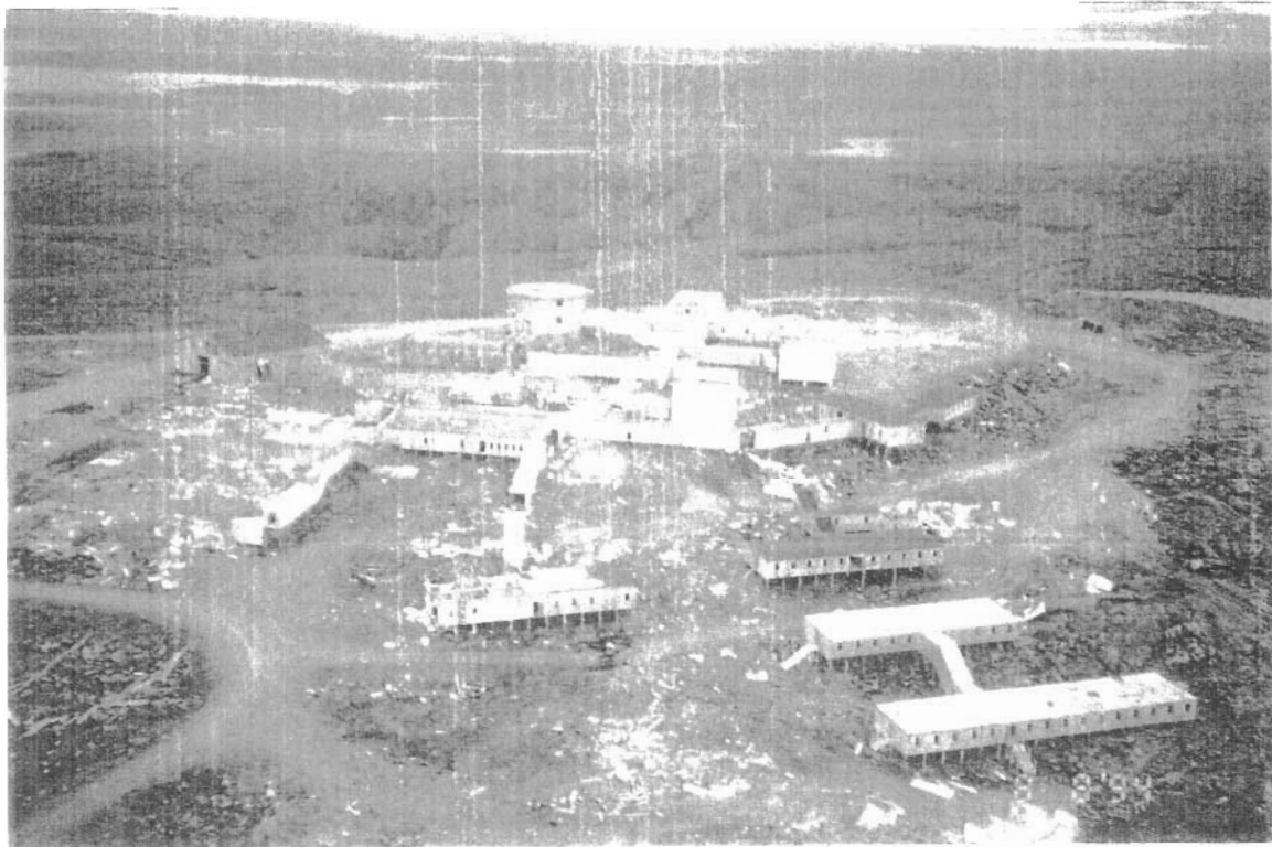
Photograph V-4: Aerial view of the Main Site at the Upper Base. Long-range radar were housed in geodesic domes formerly situated atop the rectangular towers.
