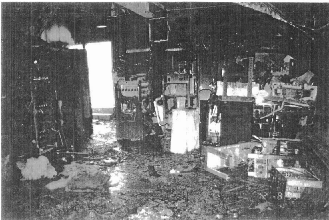
Photograph V-9: The burnt interior of Communications Building S-28 where the remains of electrical equipment were found.
