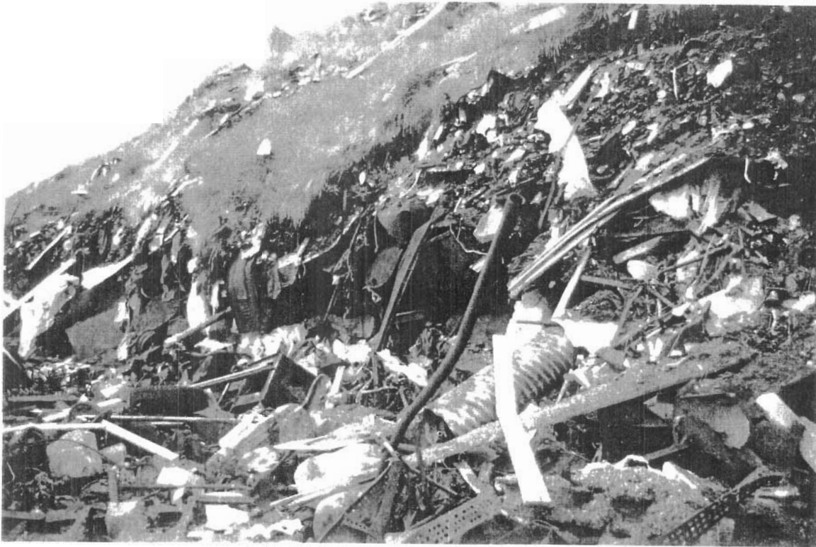
Photograph V-47: Extensive erosion of the toe of Dump Site #5 by tidal action and ice scouring.
