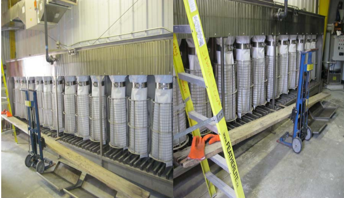
Sludge Bagging inside the WWTP
