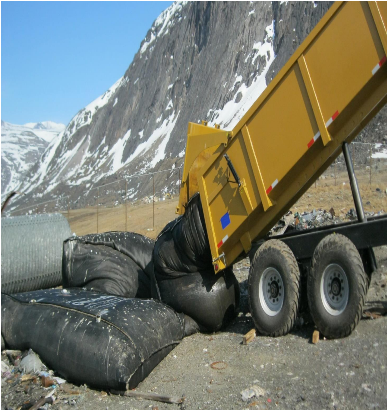
Fig:6: Geo-tube with sludge dumping at the Land Fill site
