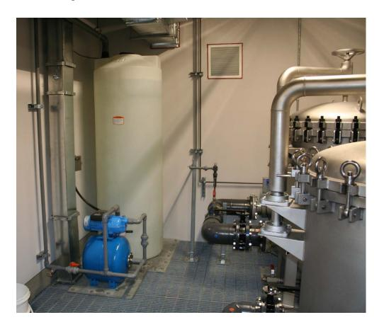
The domestic water pump is a self contain automatic pump. When water is demanded, it maintains water pressure for service sink, cleaning hose, chlorine tank filling, etc.
