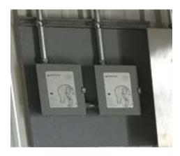
Each HTC to control: 2 heat trace cables and 3 RTD temperature sensors. There are 3 sensors per intake pipe: at 15 meters and at 30 meters.
