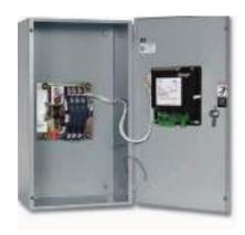
ASCO Power Transfer Switch rated 200 amperes
