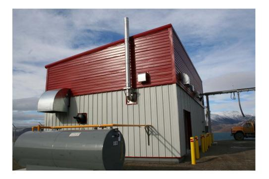
A second, smaller tank 227Liters (50 Gallon imp.) is located near the boiler, and holds enough fuel to supply the furnace and the back-up generator.
