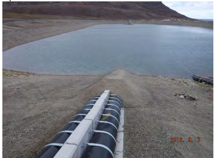
View of granular cover over intake pipes looking towards west into the reservoir
