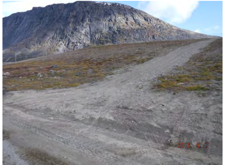
View of reservoir's northern berm exterior where erosion has been regraded/repared. View looking towards southeast.
