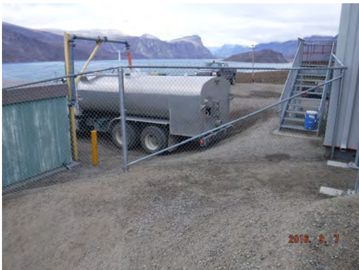
View of area adjacent to new truck fill station stairs that are being encroached on by trucks using old truck fill station. Fill to extend approximately 1 m from the stairs towards the rear of the truck in the photograph.
