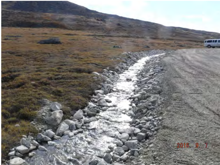
View of secondary diversion ditch along new truck turn around showing flow from pump testing. View looking towards southwest.
