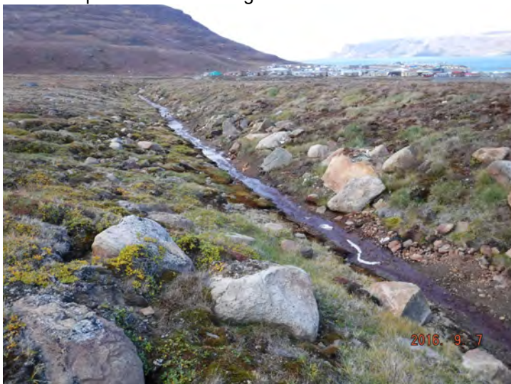
View of primary diversion ditch looking towards west showing flow of water towards the west.
