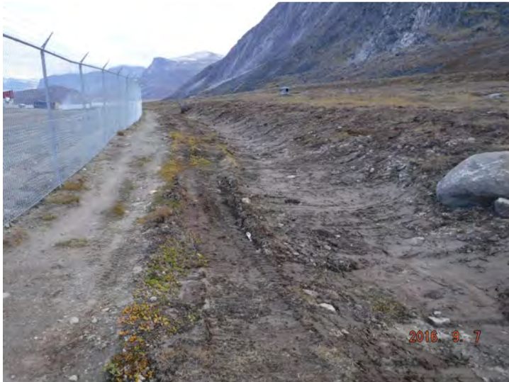
View of secondary diversion ditch, showing area that will need to be regraded by Kudlik. Kudlik to submit photograph once completed. View looking towards east.
