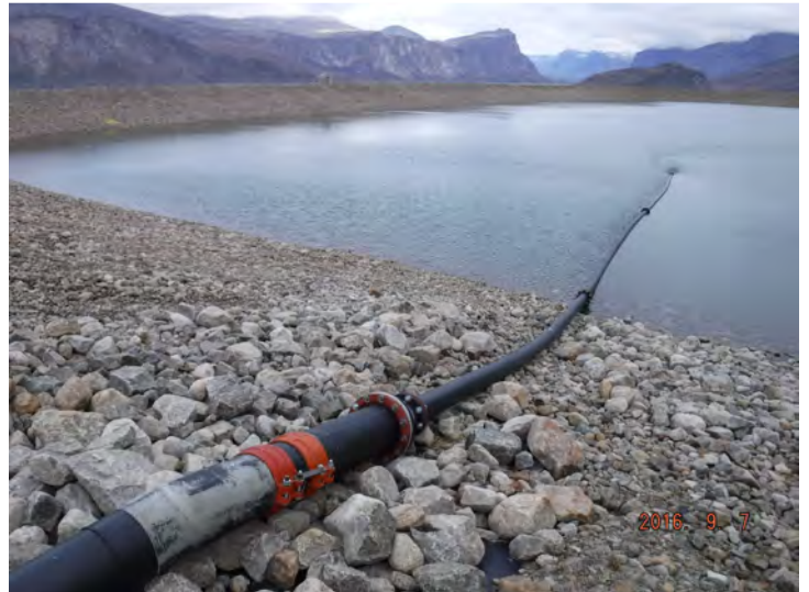
Western interior slope adjacent to filler pipe repaired with rip-rap
