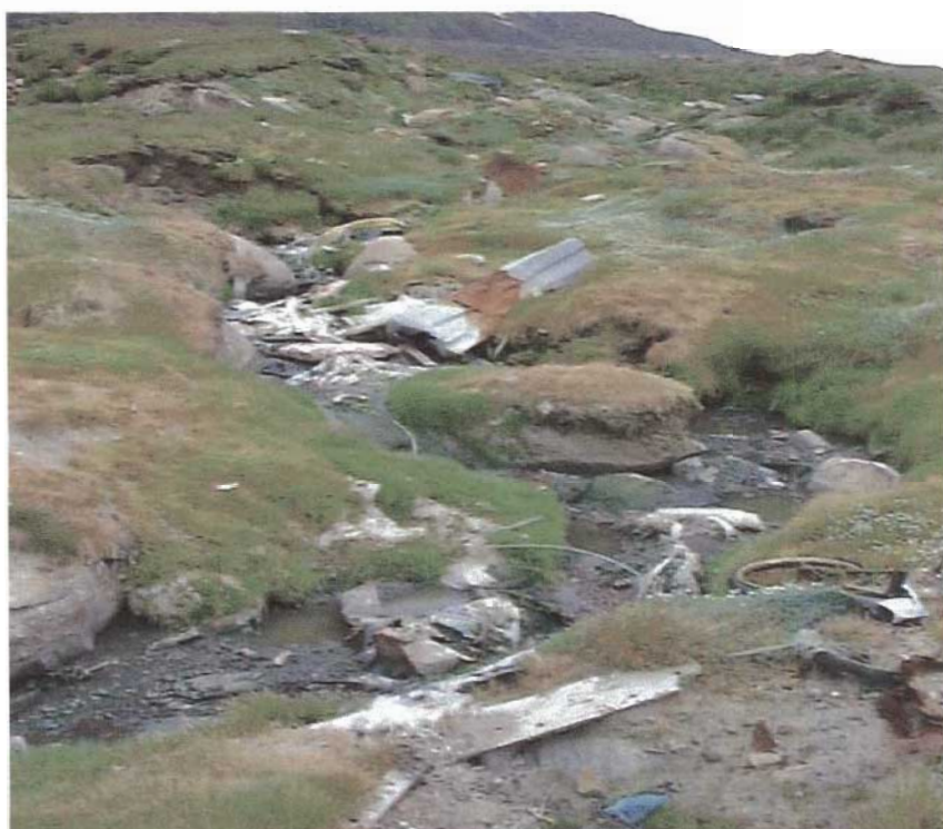
figure 3. Path of discharge from the sewage disposal facility; 2001/07/16.
