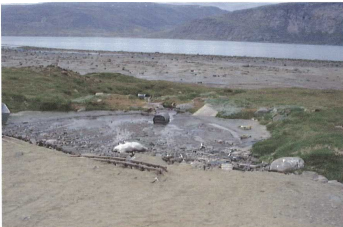
figure 2. Sewage disposal facility; 2001/07/16.
