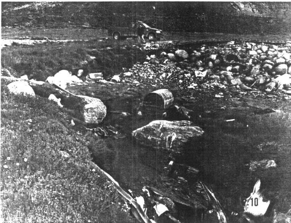
Photo # 16 Sewage lagoon; shown minuets after discharge from sewage truck. Note that little if any retention of sewage is accomplished at lagoon
