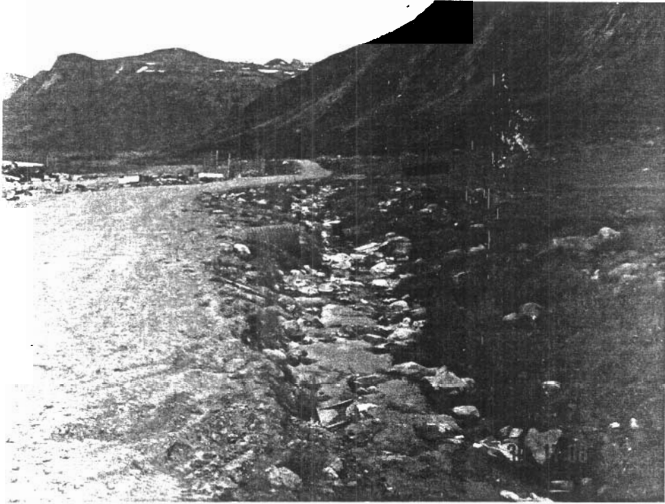
Photo # 11 Ditch across the road from solid waste disposal ground; windblown refuge shown in ditch.
