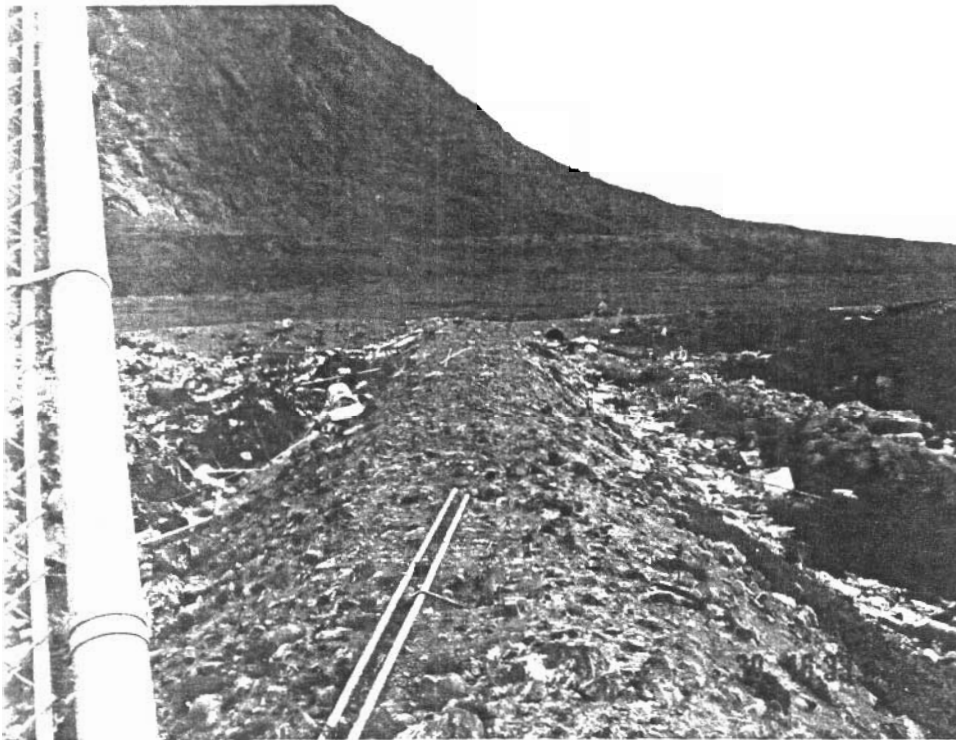
Photo # 14 Solid Waste Disposal Facility berm shown; separating creek from landfill. Fence has been damaged and is no longer in place along berm. Considerable garbage has been windblown into creek.
