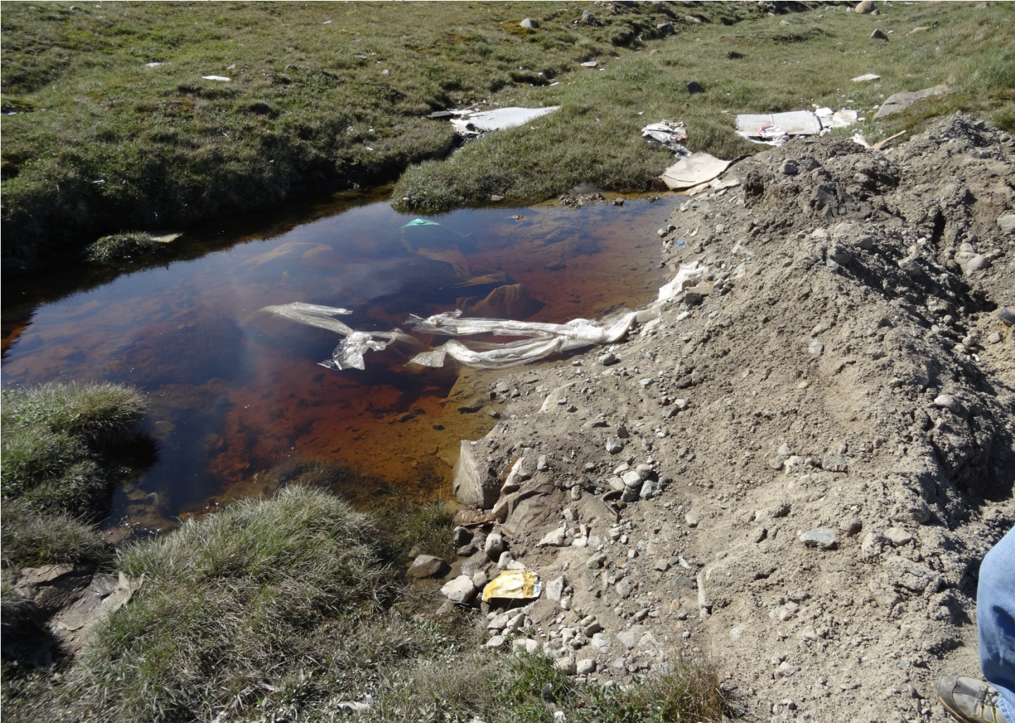
Figure B: One of three locations where water has built up behind the berms surrounding the metal storage area.
