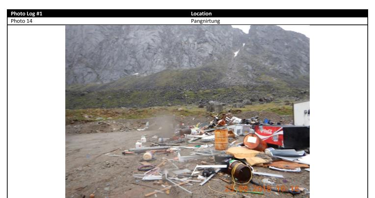
Description: Hazardous Waste in the Bulk Metals section. Waste Oil Drums, can propane tanks can be seen littered around the entrance fringes of the Bulk Metals section. Embankment appears to be working diverting water into the Solid Waste Facility.
