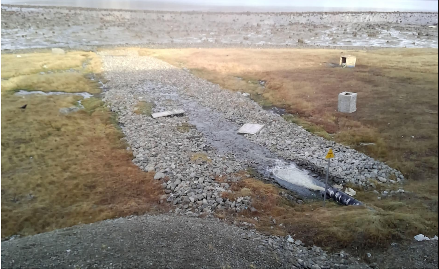
Description: Spill from within the facility. Spill drains into a sump pit in the receiving side of the waste water facility. At the time of the inspection, it was unknown if the facility was operating as intended as there was no operator, and it appears that a truck that discharged into the facility, had triggered this decant. It is unknown whether the facility was doing any treatment.
