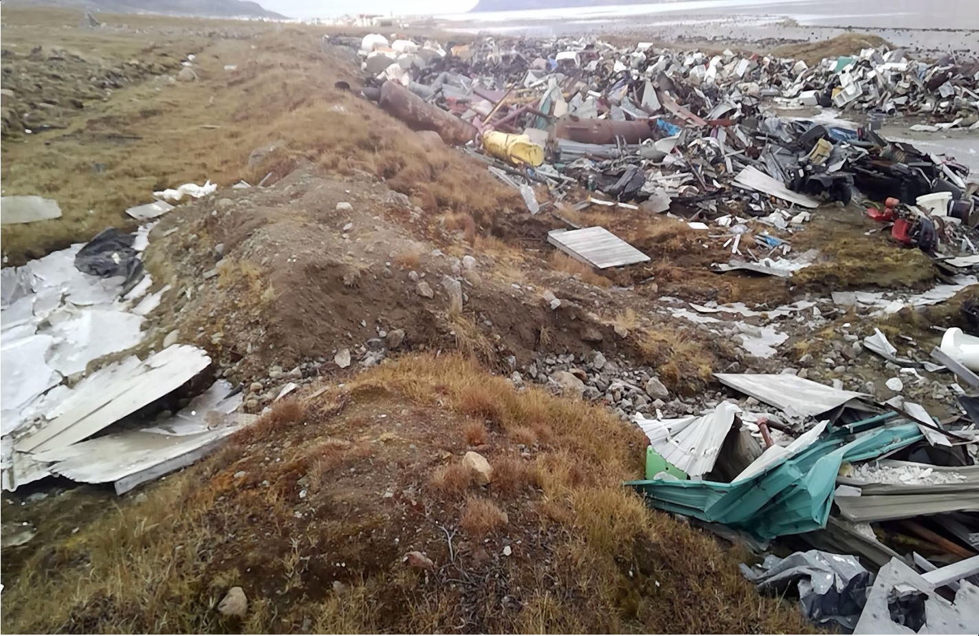
Description: Hazardous Waste in the Bulk Metals section. . A couple of parts of the walls on the East side of the Bulk Metal, and Treated Wood appear to have washed out. These washed out walls need to be repaired to ensure that no water is entering the facility, and taking waste with it as it exits the facility.
