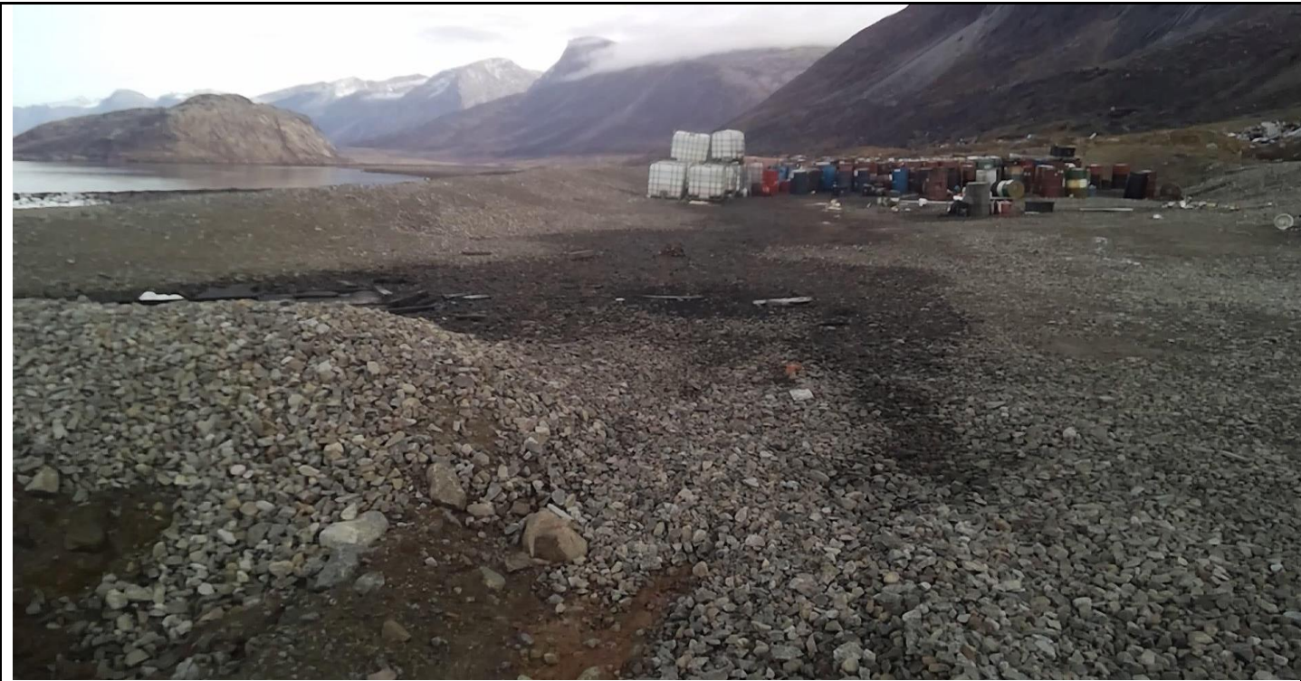
Description: The drums from Spill Report 2019-244, placed into a non-engineered secondary containment. New spill migrating towards the opening of the non-engineered berm for hazardous waste. A spill report should be generated for this spill, and mitigate the migration of it.
