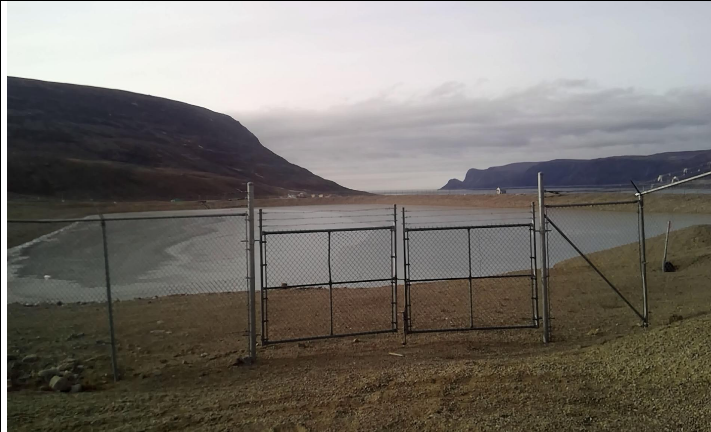
Description: Water Reservoir capacity is 12,000m³ in the summer, and taking in considerations for the 1.8 metres of ice 71,000m³ in winter.
