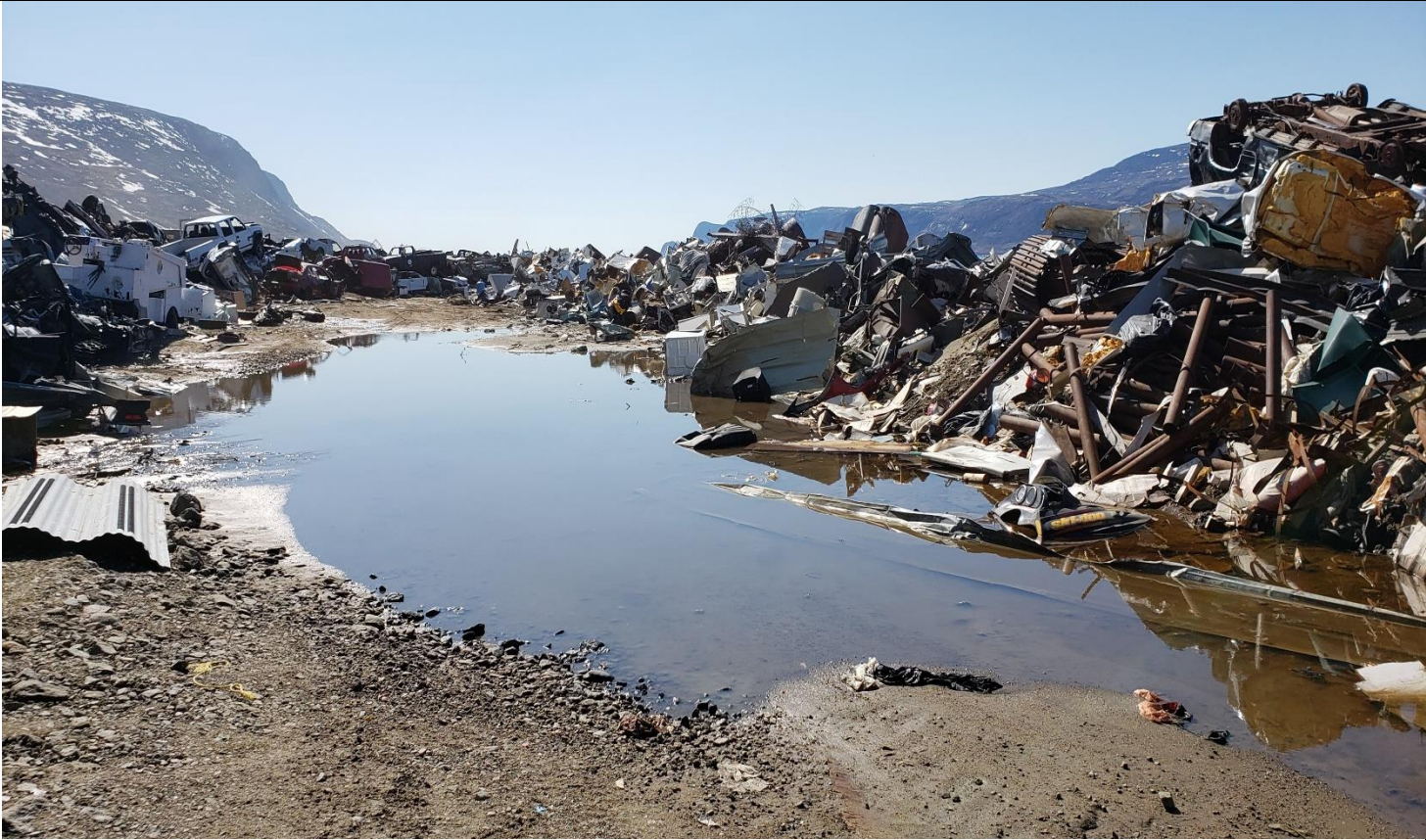
Description: Bulk Metals section. East Corner of the Bulk Metals Facility. The wall to divert water from entering the facility has washed away. The washed away wall, allows surface water to move through one of three hazardous waste facilities.
