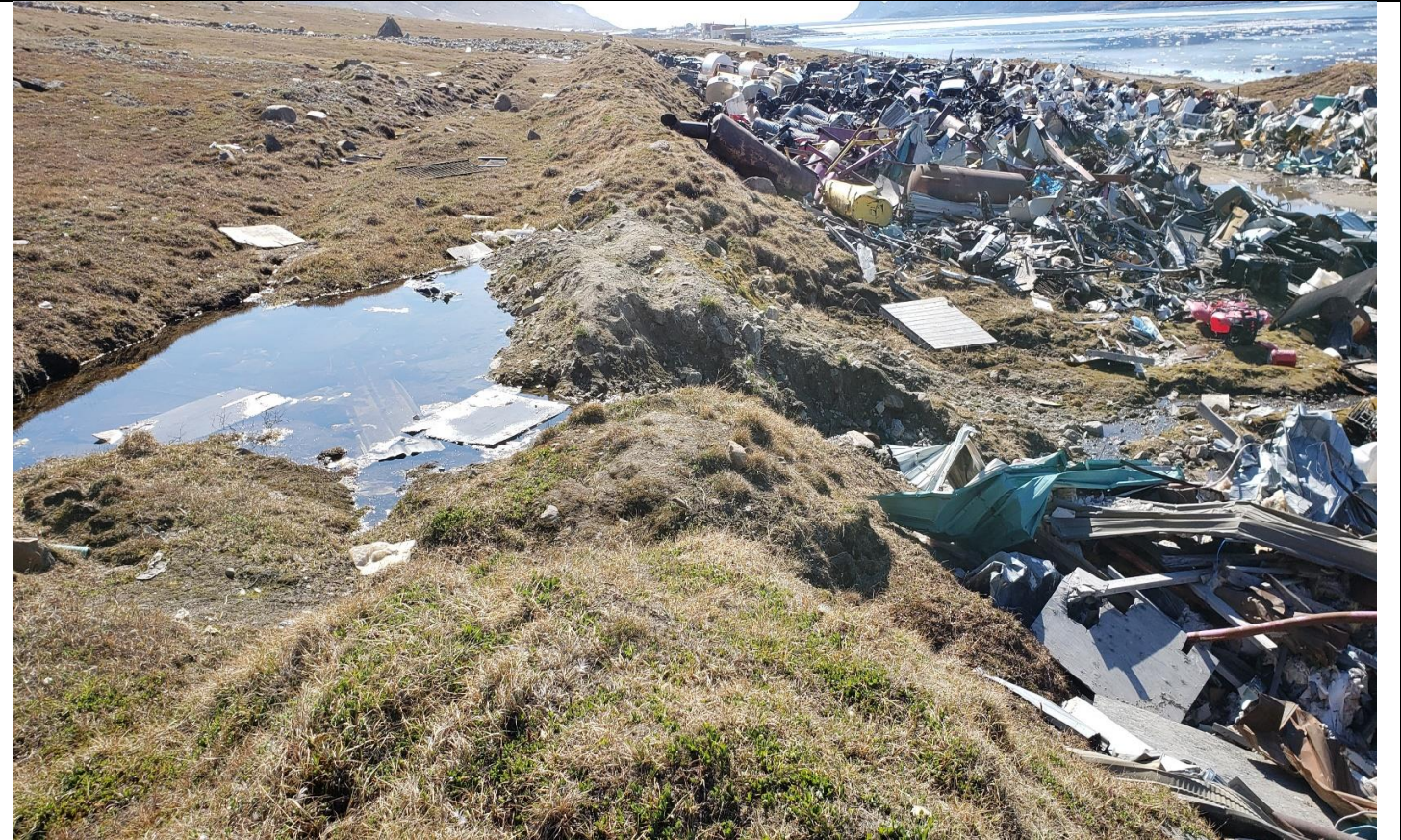
Description: Hazardous Waste in the Bulk Metals section. A couple of parts of the walls on the East side of the Bulk Metal appear to have washed out. These washed out walls need to be repaired to ensure that no water is entering the facility, and taking waste with it as it exits the facility.
