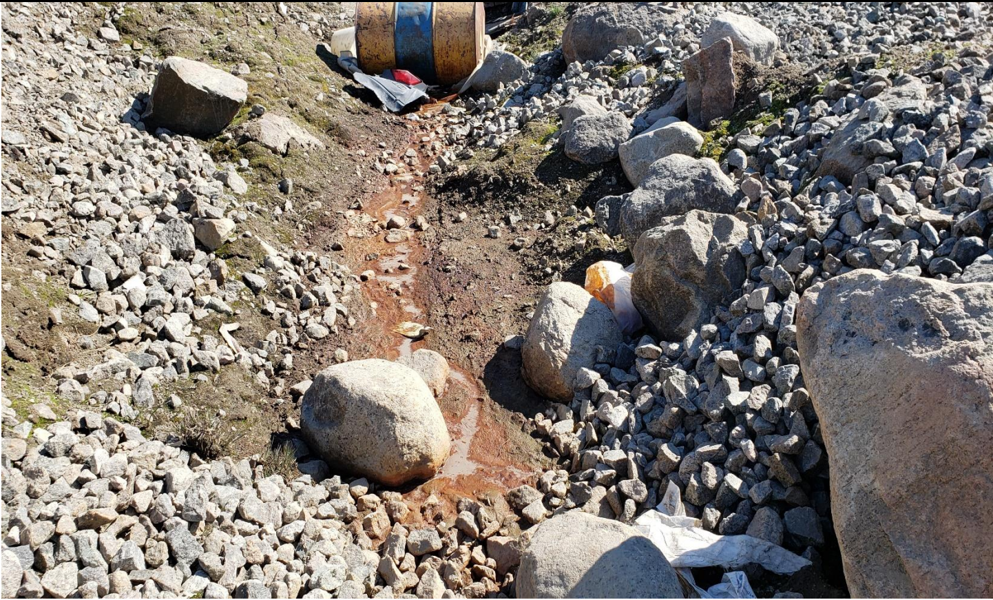
Description: subsurface water drainage exposed and migrating out of non-engineered berm used to house the hazardous waste. A drum is situated in the drainage ditch, and new spill can be observed migrating towards the drainage ditch.
