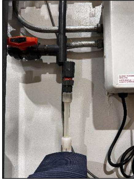
Figure 17: Defoamer ½" PVC Replacement from Pump Discharge to Tee
