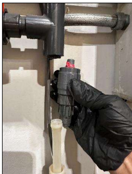
Figure 15: Defoamer Injection Quill and Cracked Piping
