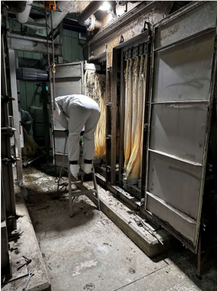
Inspecting Existing Membranes (1)
