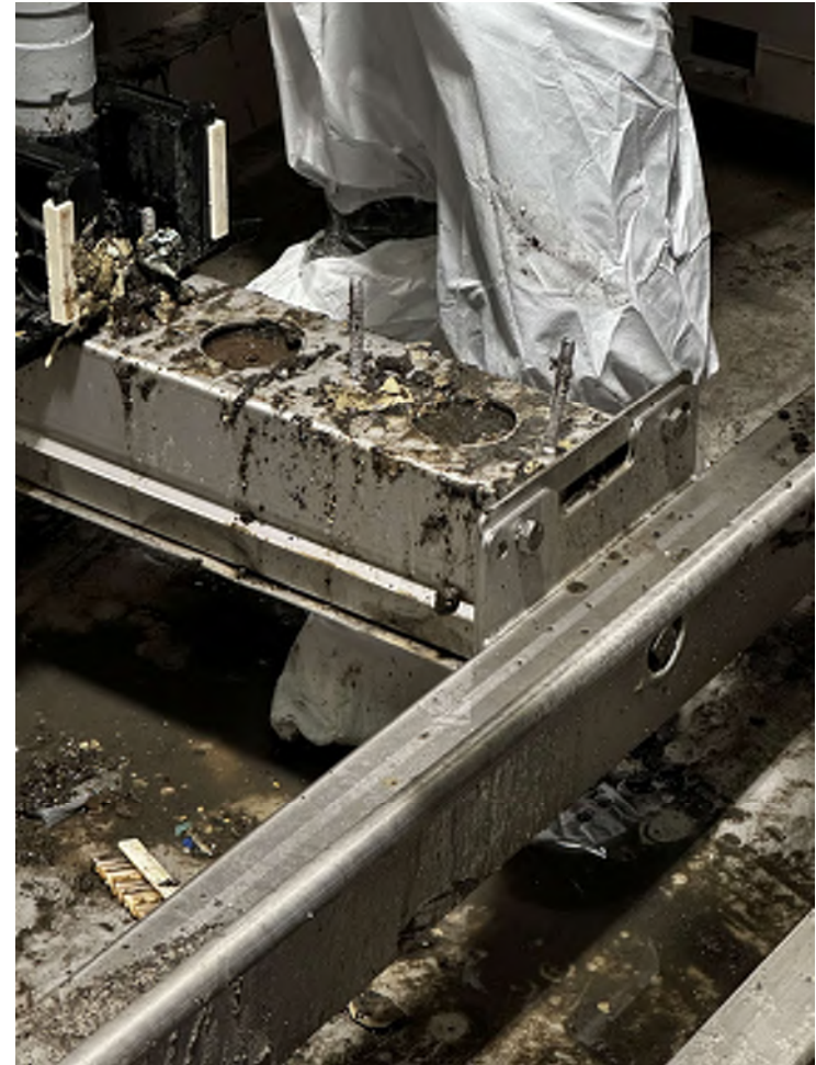
Removing Existing Air Scour Piping and Cassettes (4)
