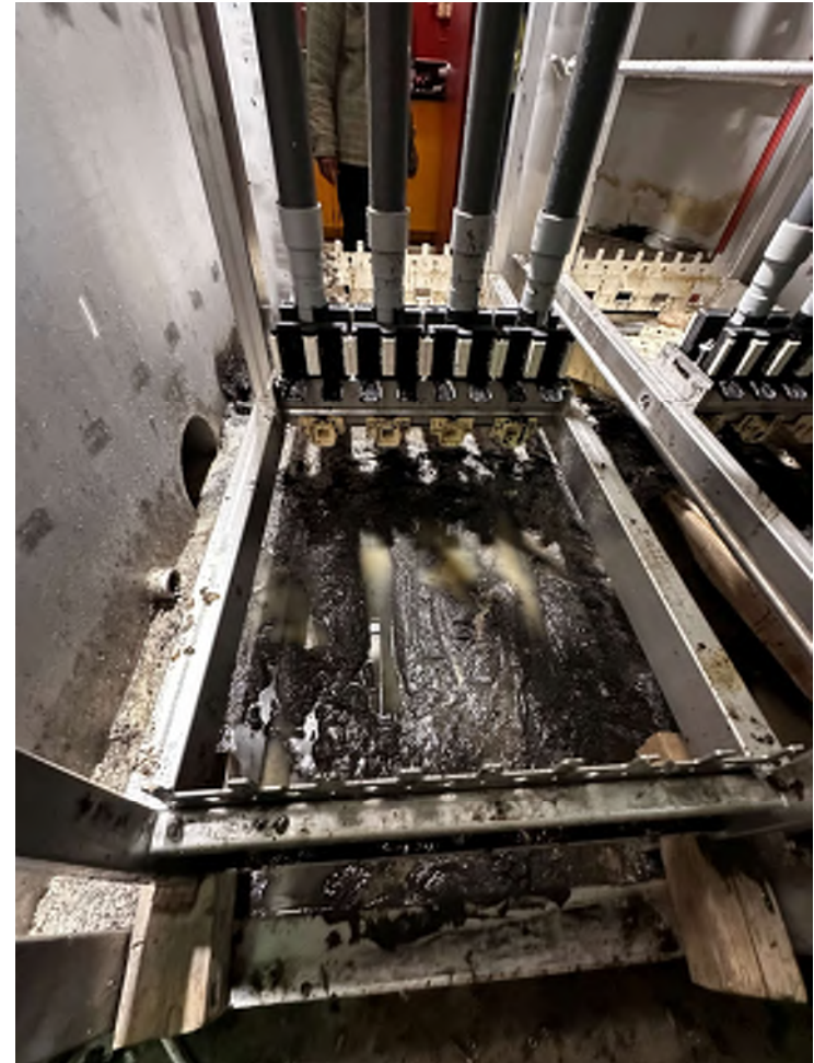
Membrane Tank Sludge Accumulation (0)
