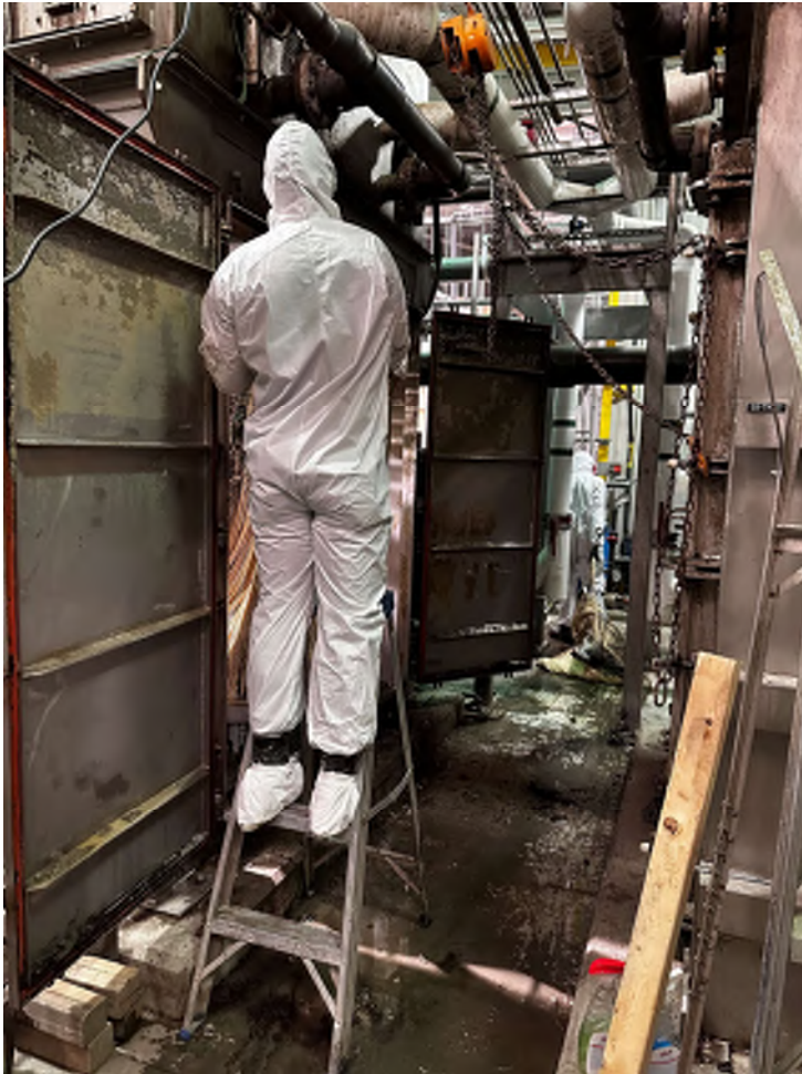
Removing Existing Membrane Module (1)
