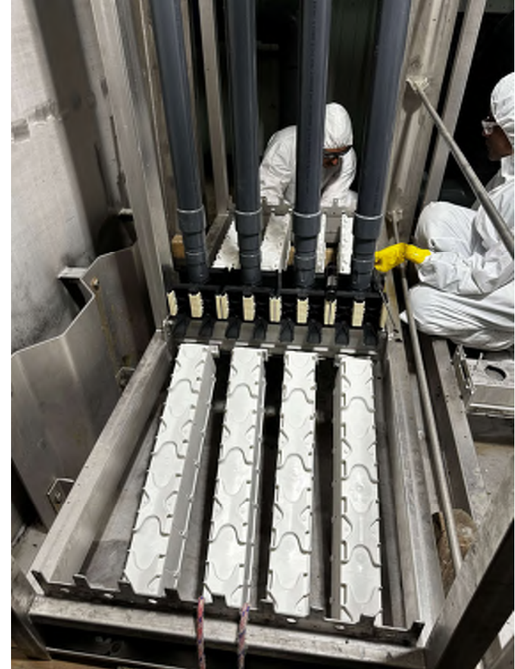
Installing New Air Scour Piping (1)
