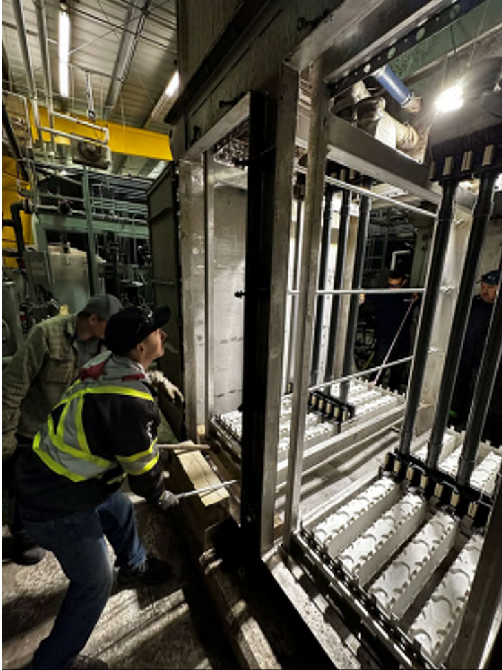
Installing New Air Scour Piping (4)
