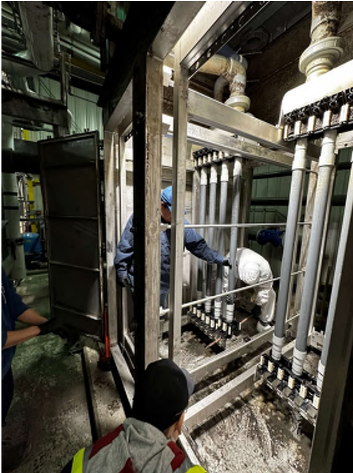
Removing Existing Air Scour Piping and Cassettes (1)
