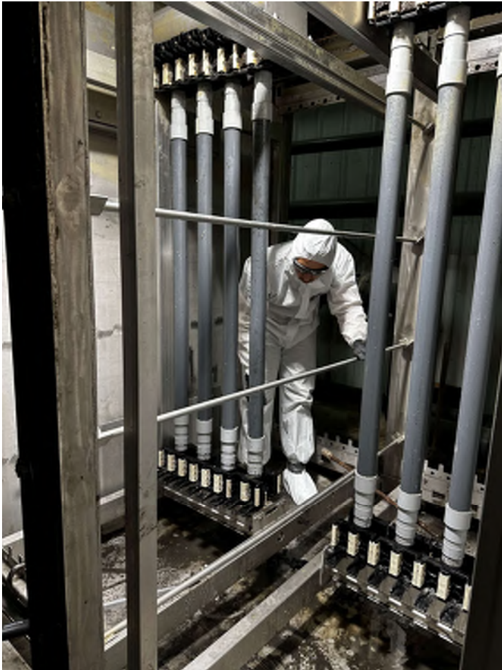
Removing Existing Air Scour Piping and Cassettes (3)
