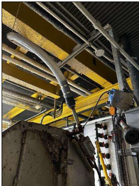
Figure 8: Cracked Solenoid Valve for Drum Screen Wash
