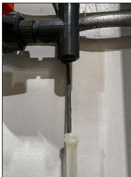
Figure 15: Defoamer Injection Quill and Cracked Piping
