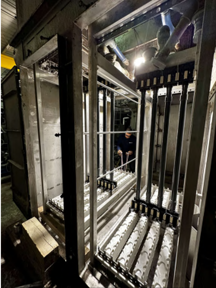
Installing New Air Scour Piping (2)
