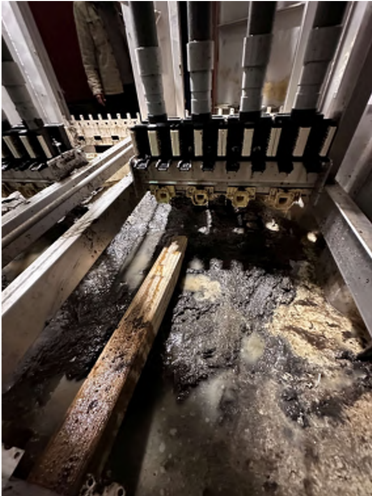
Membrane Tank Sludge Accumulation (1)
