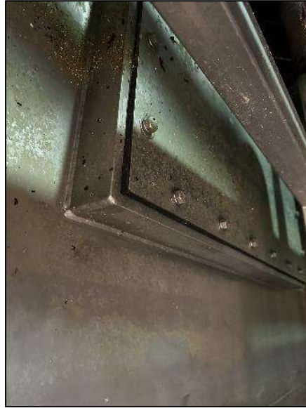
Figure 33: Tank 1 - Overflow Weir
