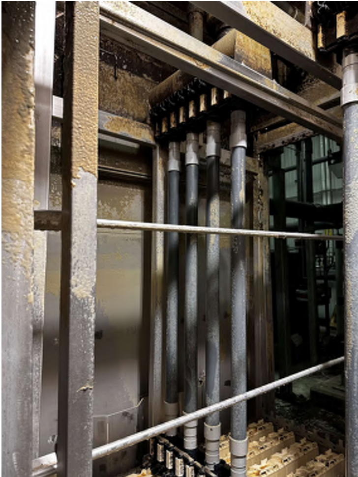
Removing Existing Air Scour Piping and Cassettes (5)
