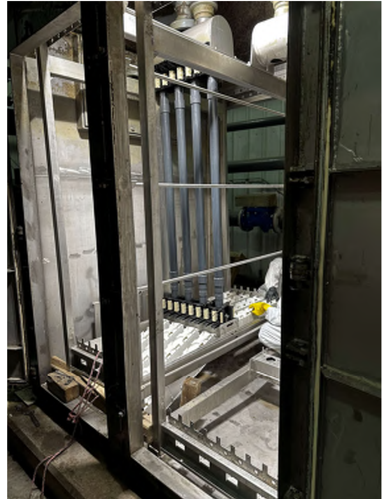
Installing New Air Scour Piping (0)
