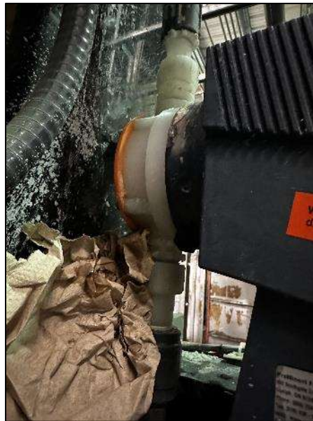
Figure 39: Sodium Hypo Pump Leak behind Pump Diaphragm
