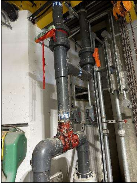
Figure 6: Cracked 4" PVC Screened Pump Discharge Tee
