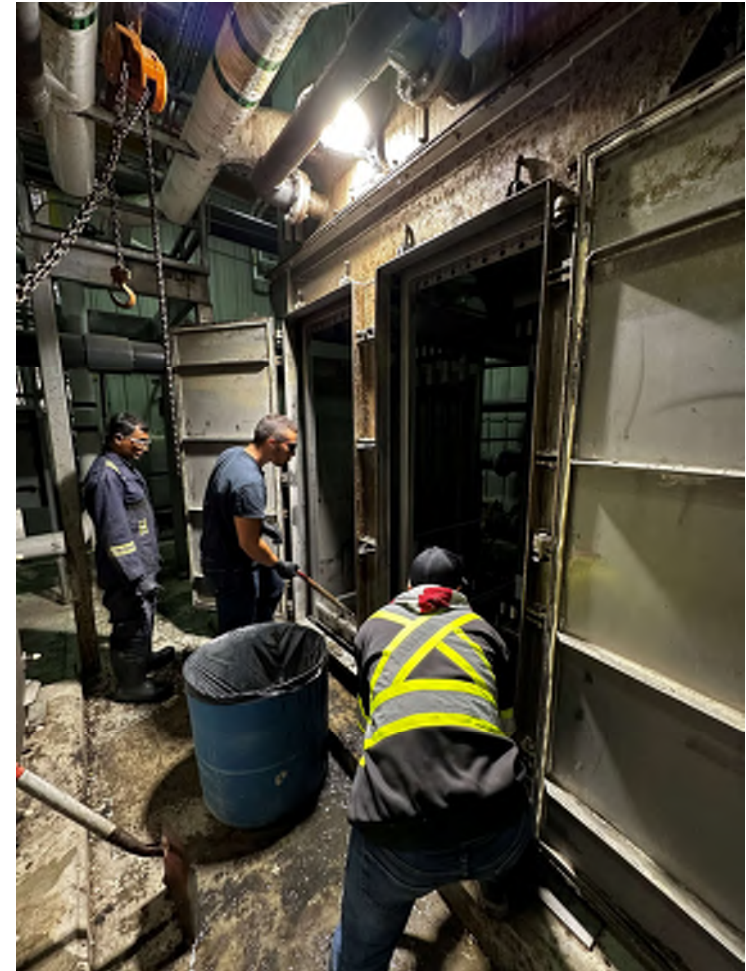
Clearing Membrane Tank of Accumulated Sludge
