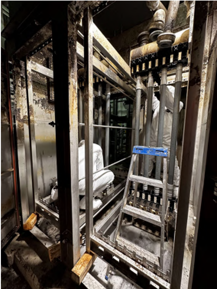
Installing New Air Scour Piping (6)
