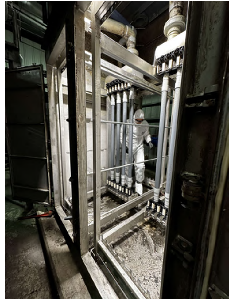
Removing Existing Air Scour Piping and Cassettes (2)
