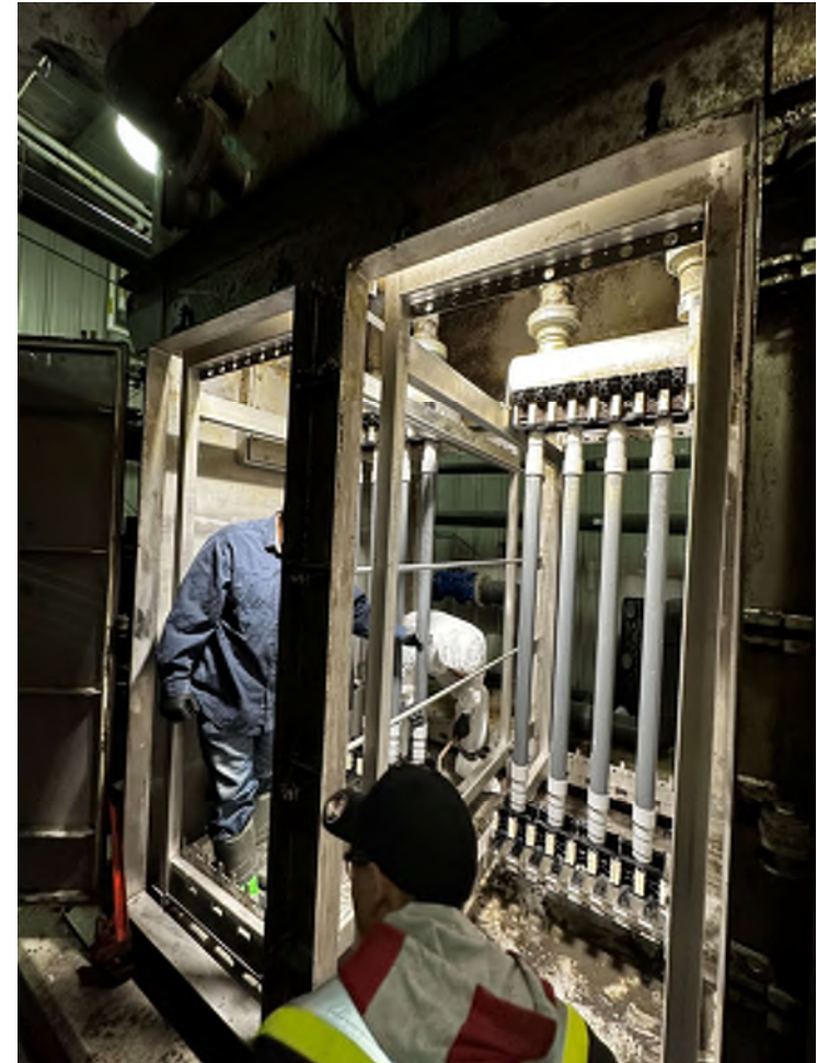
Removing Existing Air Scour Piping and Cassettes (0)
