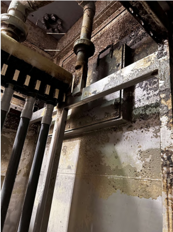
Membrane Tank Internal Air Piping
