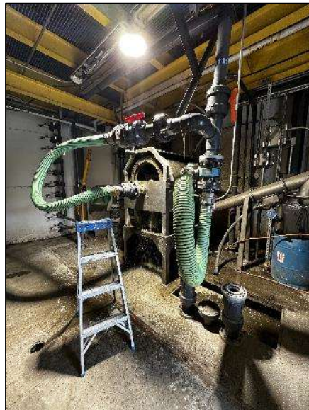
Figure 14: Existing Raw Sewage Pump/Sump
