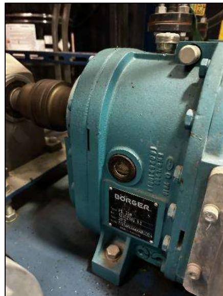
Figure 38: Permeate Pump Oil Change
