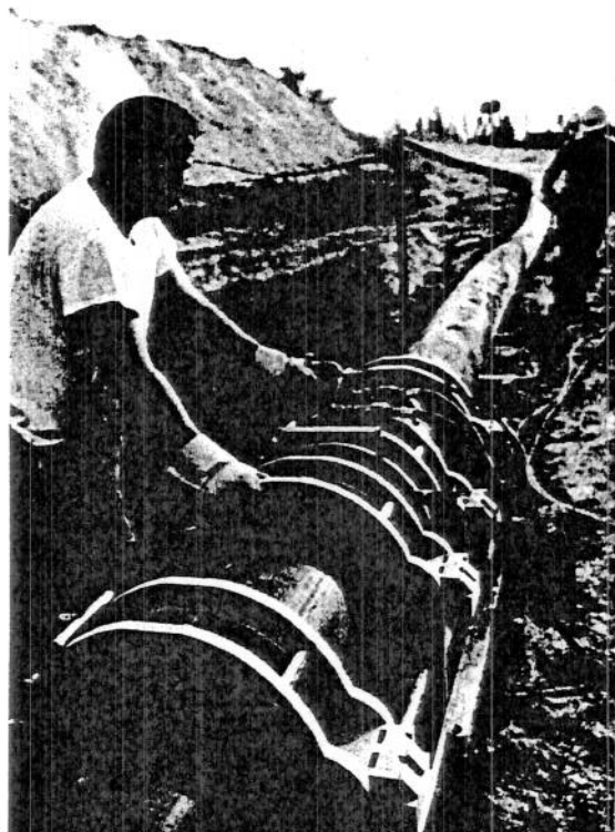
Techline HDPE pipe sections are joined by portable butt welding equipment.
