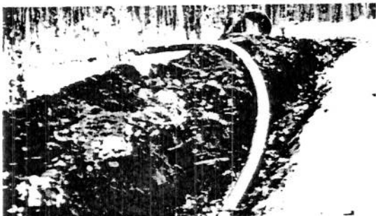
Flexible Techline® easily handled in long butt fused lengths.
