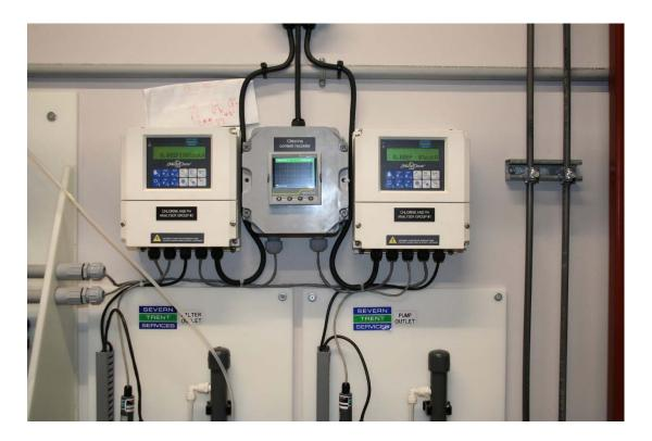
The two key component are the chlorine probes and PH probes.
