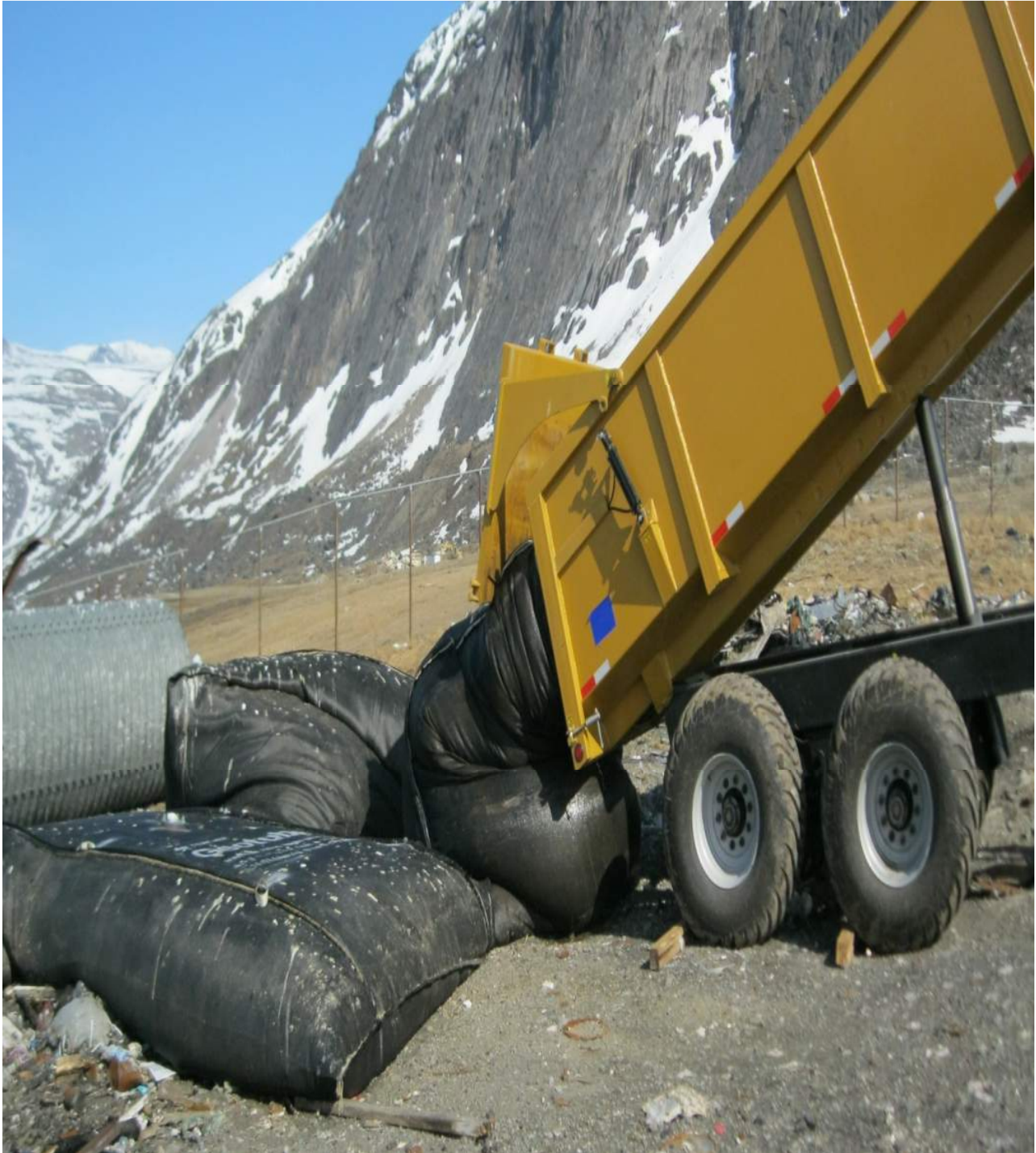
Figure 9: Geo-tube with Sludge Dumping at the Landfill Site
