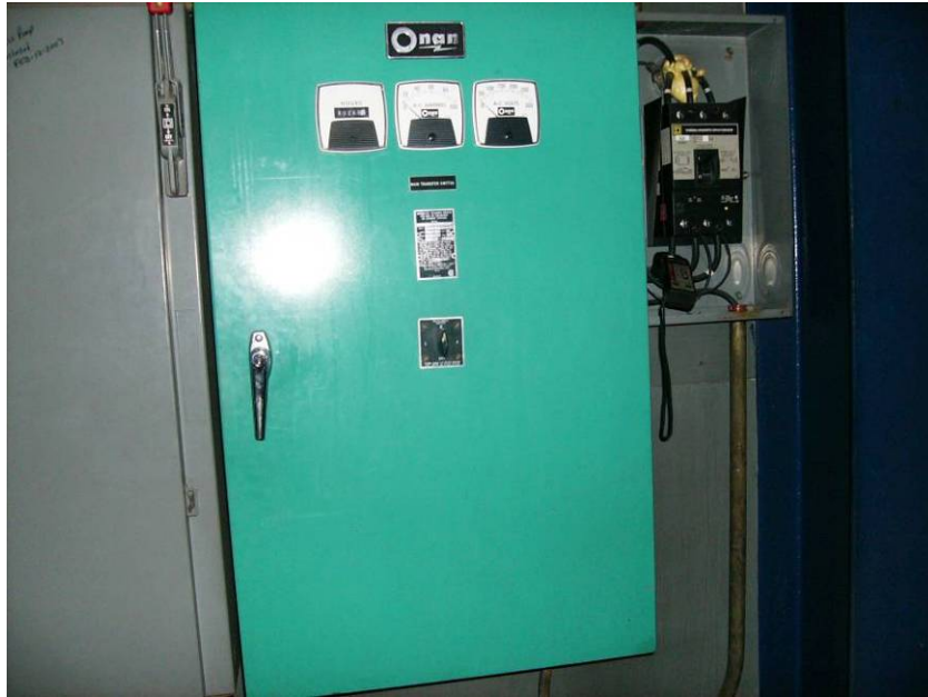
Photograph No. 7.2.2.a - 120/208 Volt Secondary Distribution: Transfer Switch and Main Service Breaker
