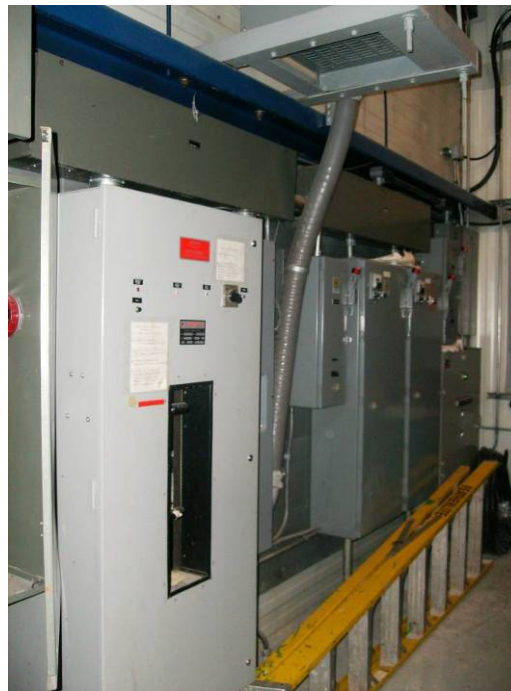
Photograph No. 7.1.2.d - 120/208 Volt Secondary Distribution: Automatic Transfer Switch and Starters
