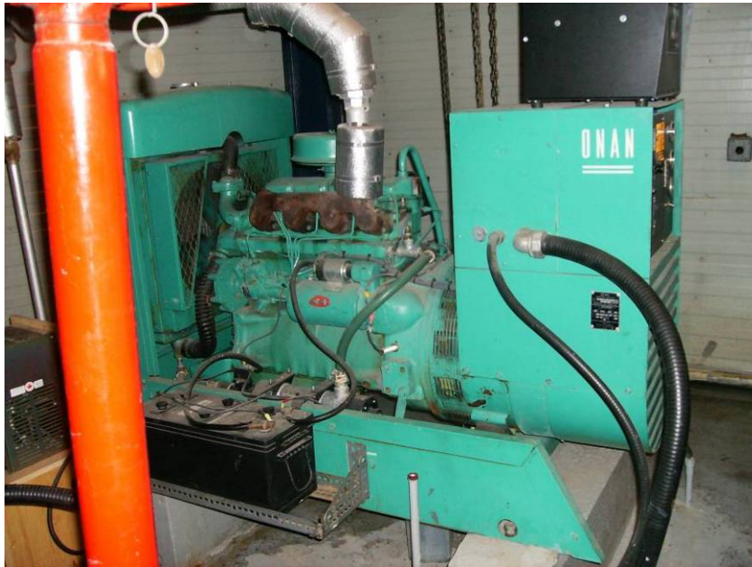
Photograph No. 7.1.4.a : Emergency Power – 100 kW – 120/208 volt Generator
