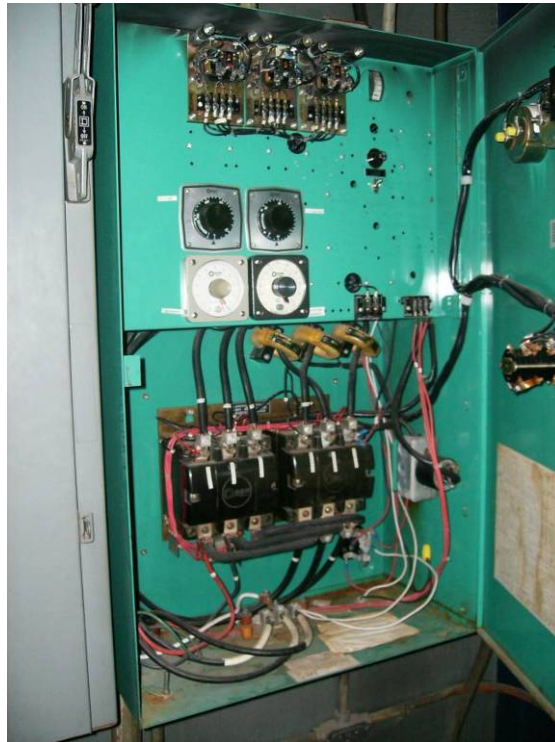
Photograph No. 7.2.4.a - Emergency Power – Transfer Switch
