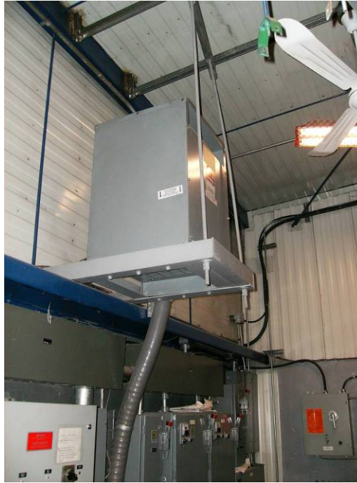
Photograph No. 7.1.2.i - 120/208 Volt Secondary Distribution: Main Water Supply Heat Tracing 50 kVA 208 to 600 volt Transformer
