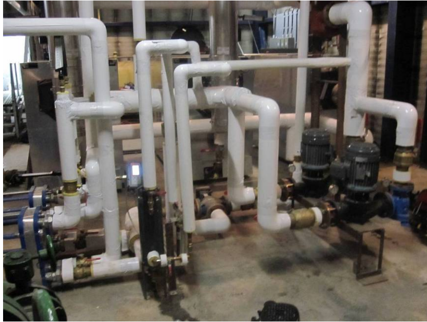
Picture 6.2.4.2.a – Water Treatment Plant hot water pumps and heat exchangers
