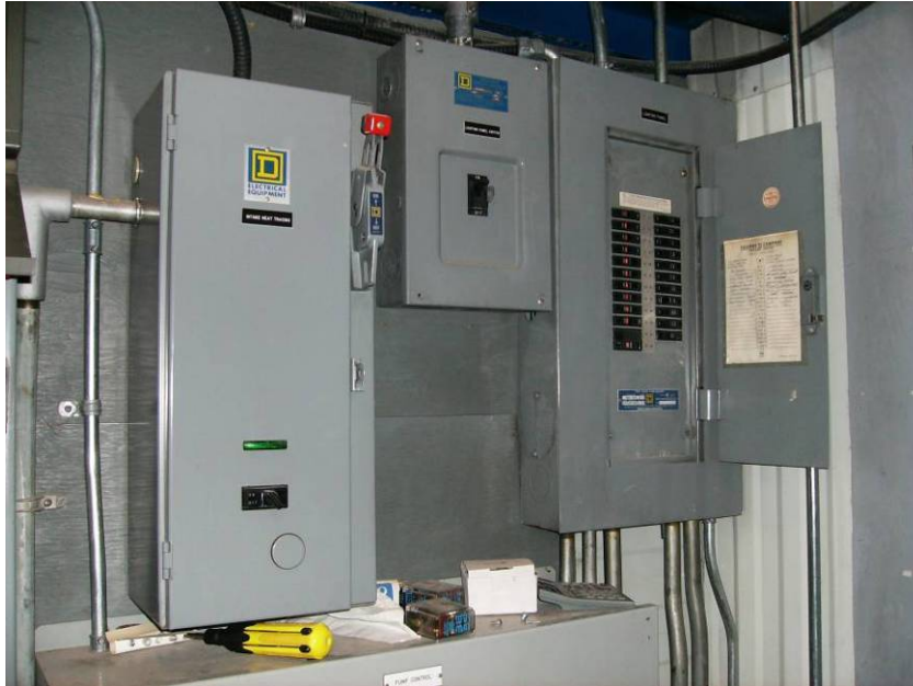
Photograph No. 7.1.2.g - 120/208 Volt Secondary Distribution: Lake feed heat tracing, Main Breaker and Lighting Panel
