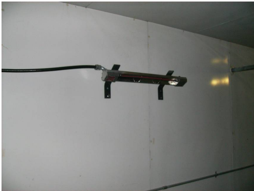
Picture 6.3.3.a – Macerator radiant heater
