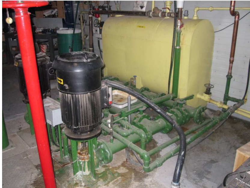
Picture 6.1.3.4.a – Diesel day tank and potable water transfer pumps
