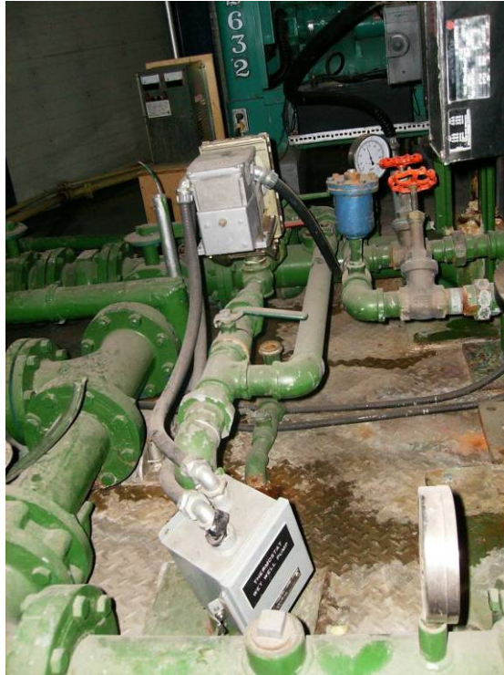
Photograph No. 7.1.6.c - Instrumentation Control and Annunciation: Redundant and Unused piping and old control valve
