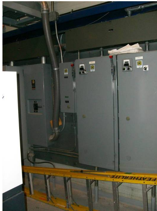
Photograph No. 7.1.2.f - 120/208 Volt Secondary Distribution: Main Feed Pump Starters and Heat Tracing Supply Contactor
