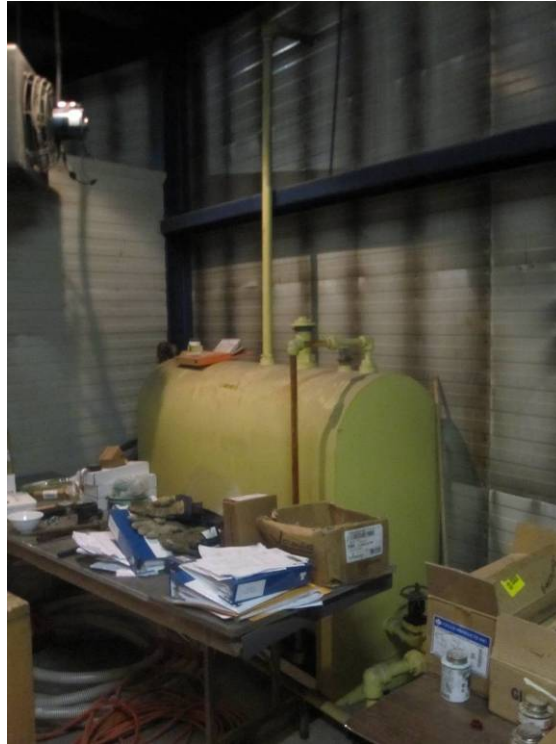
Picture 6.2.3.3.a – Water Treatment Plant diesel fuel day tank
