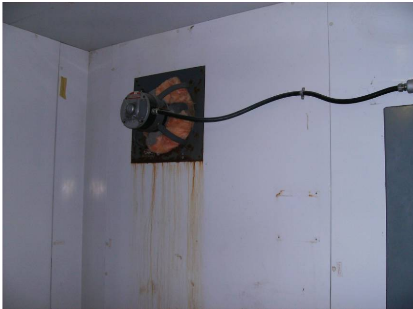
Picture 6.3.2.a – Macerator de-commissioned exhaust fan
