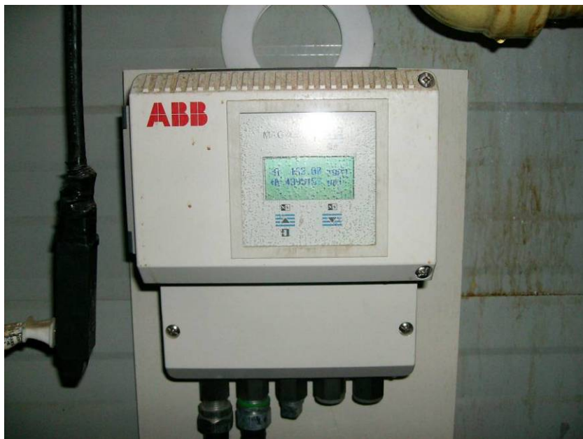
Photograph No. 7.1.6.b - Instrumentation Control and Annunciation: Flow Meter
