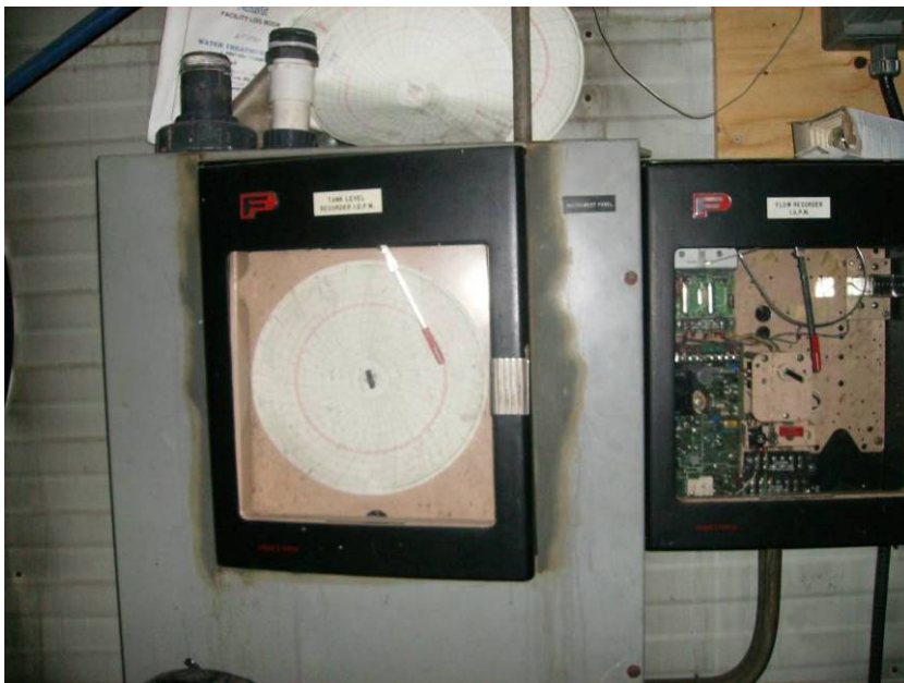
Photograph No. 7.2.6.b - Instrumentation Control and Annunciation: Consumption Chart Recorder
