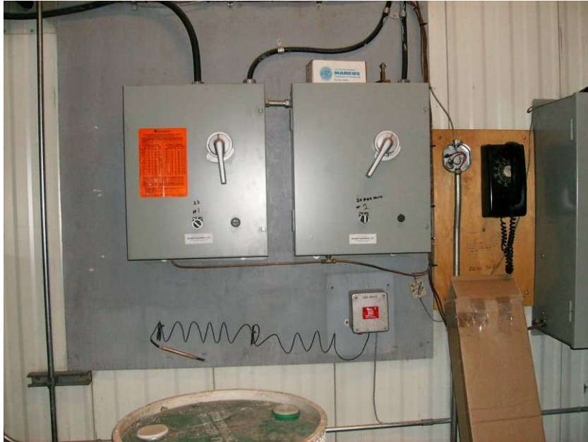
Photograph No. 7.1.3.a – Jockey Pump - Pump P1 Starter
