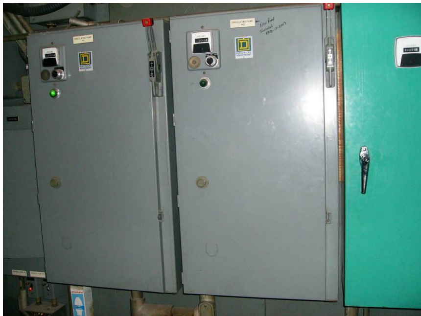
Photograph No. 7.2.3.a - Pump 1 & 2 Starters
