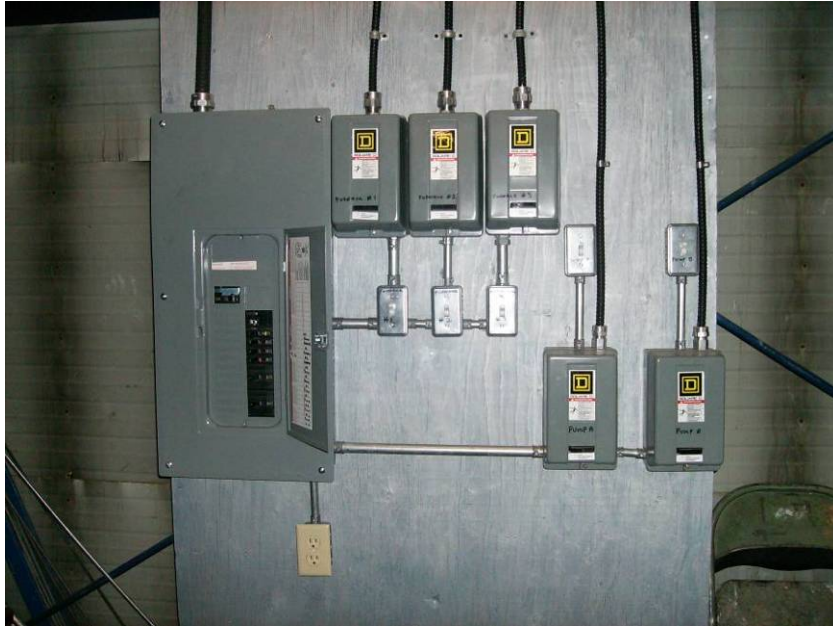
Photograph No. 7.2.2.c - Boiler Distribution: New Boiler Panel and Control Contactors
