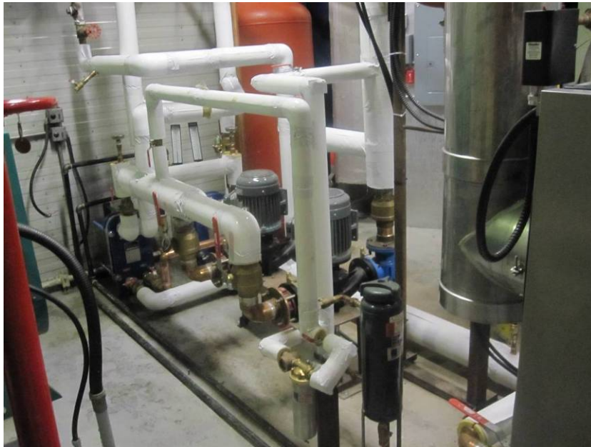
Picture 6.1.4.3.a – Char Lake hot water pumps and heat exchangers
