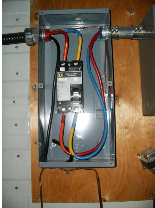
Photograph No. 7.1.2.k - Secondary Distribution Equipment, Starters, Heat Tracing: Heat Tracing 7 Amp 2 Pole Breaker
