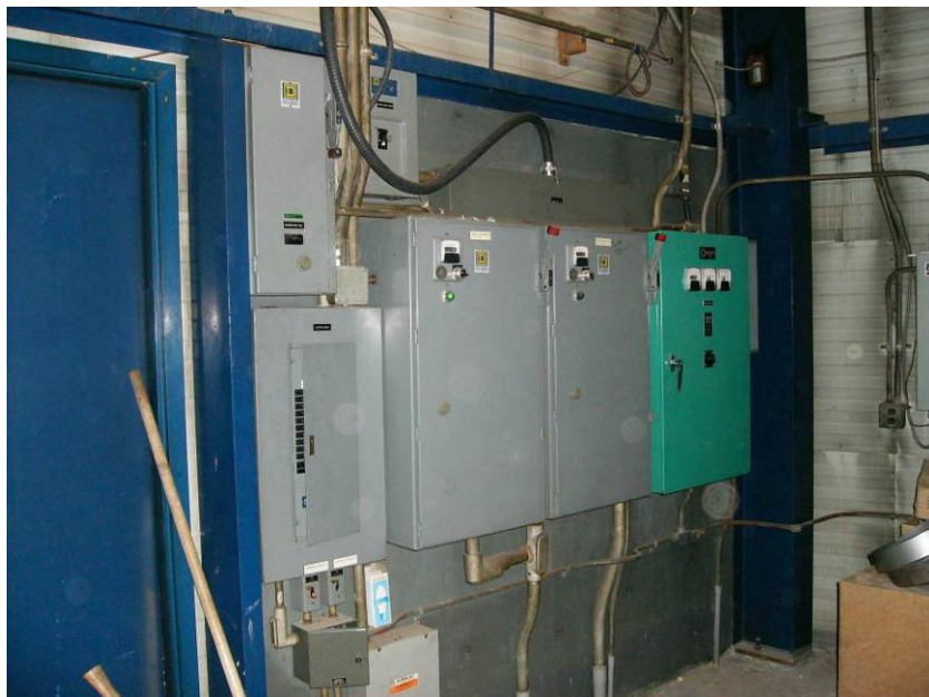
Photograph No. 7.2.2.b - 120/208 Volt Secondary Distribution: Branch Circuit Panel, Motor Starters and Transfer Switch
