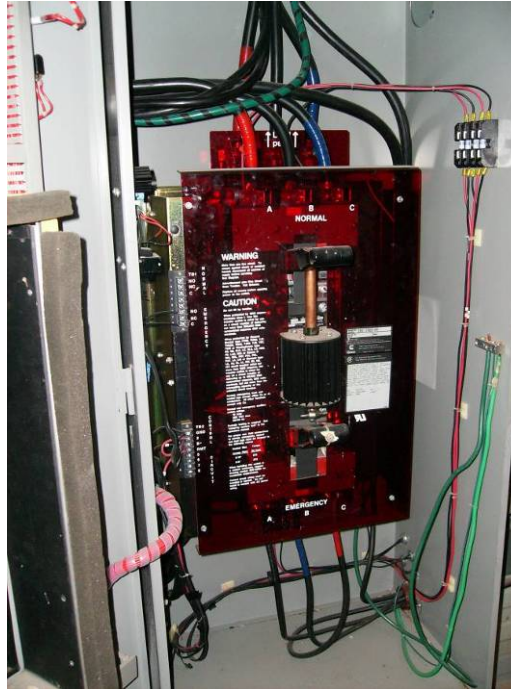
Photograph No. 7.1.2.c - 120/208 Volt Secondary Distribution: Automatic Transfer Switch
