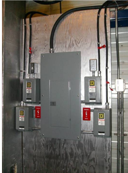
Photograph No. 7.1.2.e - 120/208 Volt Secondary Distribution: Boiler System Panel and Contactors
