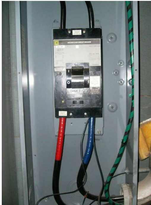
Photograph No. 7.1.2.j - 120/208 Volt Secondary Distribution: 300 Amp Feeder Breaker for Heat Tracing Transformer
