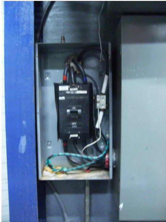
Photograph No. 7.1.2.a - 120/208 Volt Secondary Distribution: Main Service Breaker
