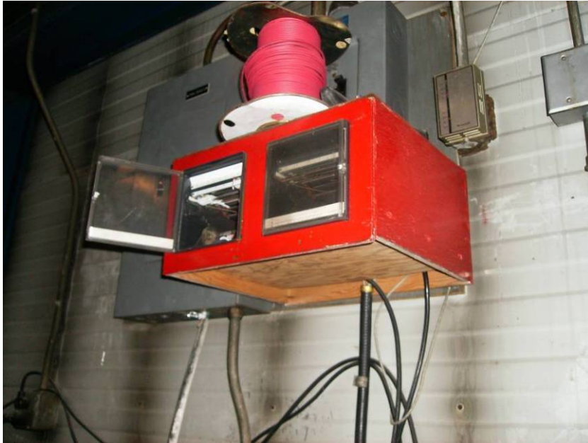
Photograph No. 7.2.6.c - Instrumentation Control and Annunciation: Temperature Monitoring Unit
