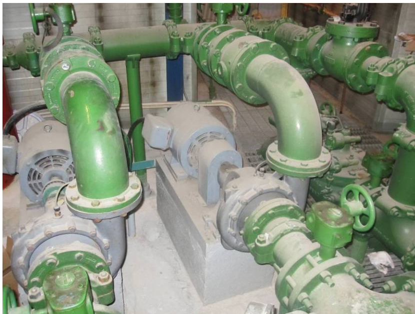
Picture 6.2.2.1.a – Water Treatment Plant circulating pumps
