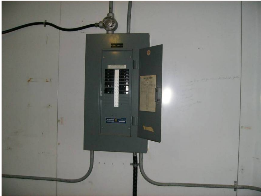
Photograph No. 7.3.1.a – Macerator: Branch Circuit Power Panel
