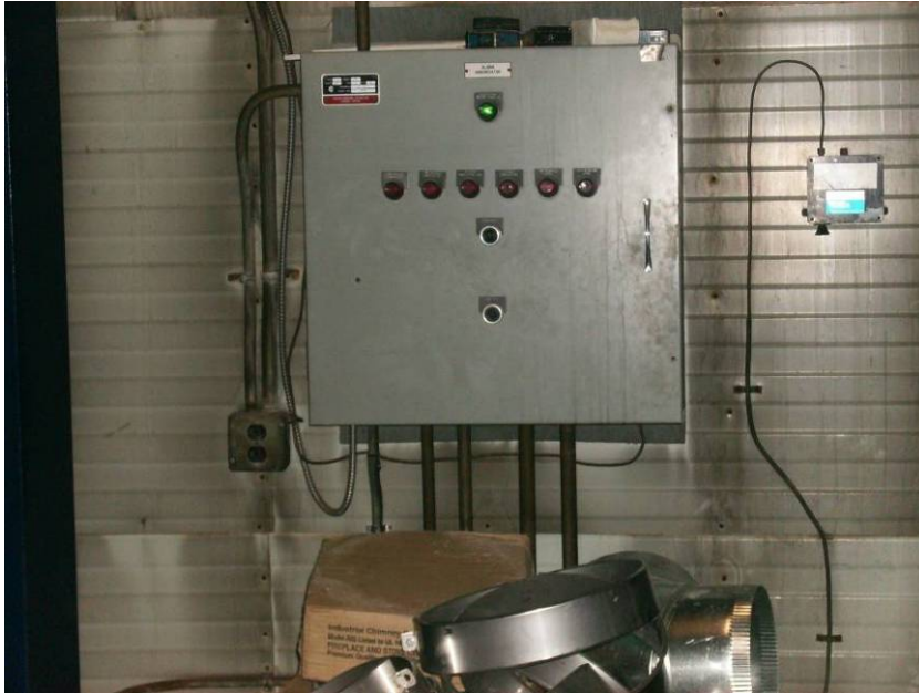
Photograph No. 7.2.6.a - Instrumentation Control and Annunciation
