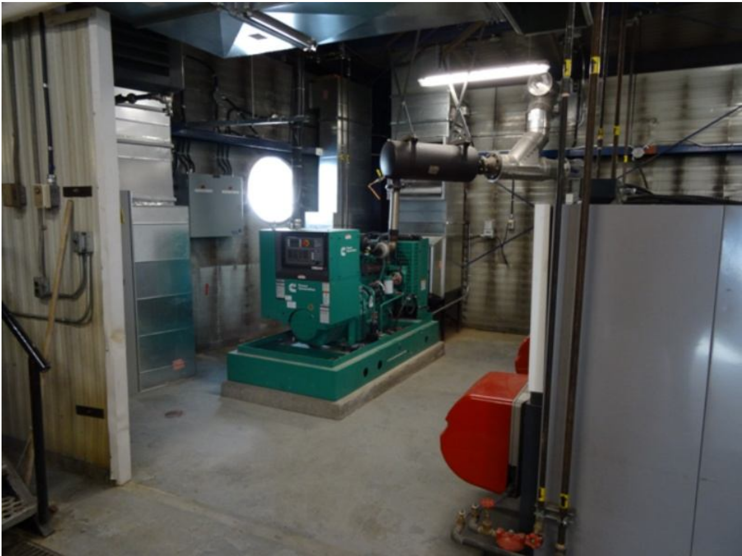
Figure 5 Backup generator at Holding tank on Signal Hill
