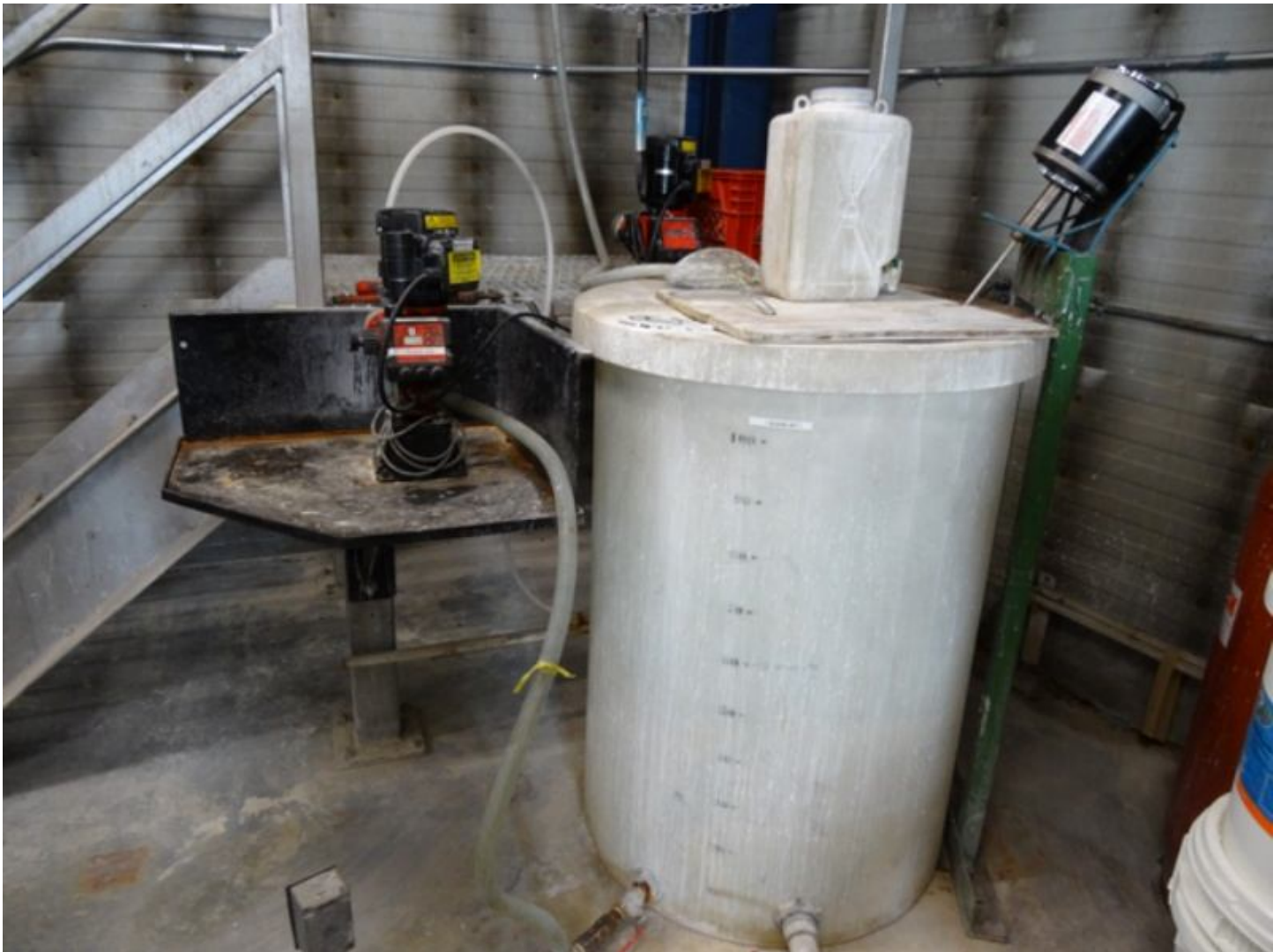
Figure 3 Chlorine mixing tank (empty) at Holding tank on signal hill - Day of Inspection
