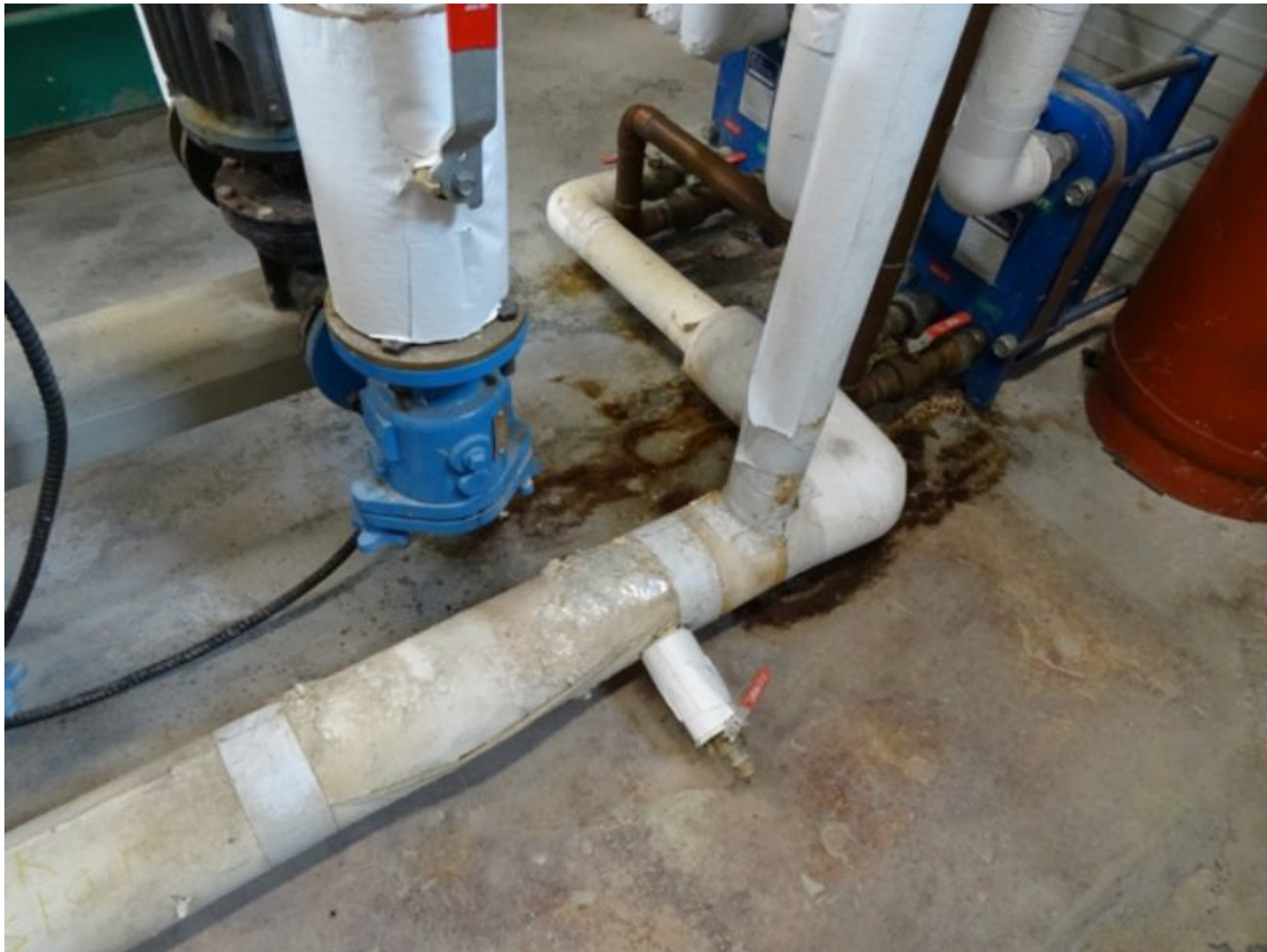
Figure 7 leaks on floor in pumping station on Signal Hill
