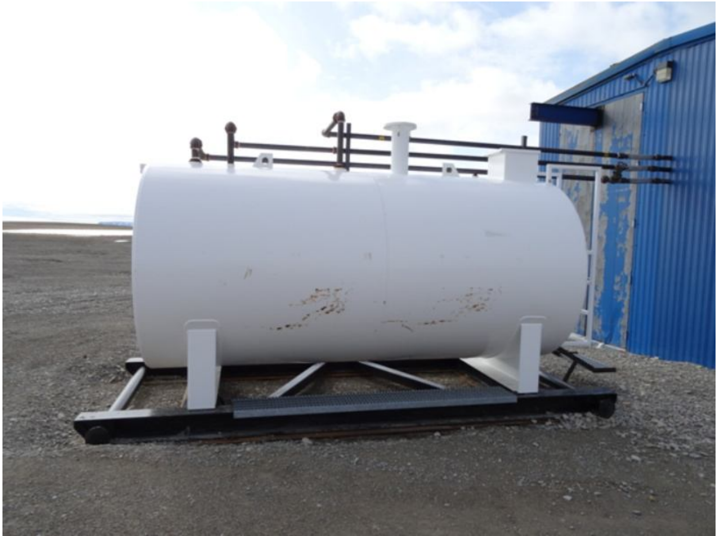
Figure 1 New double walled tank outside pump station at Char Lake
