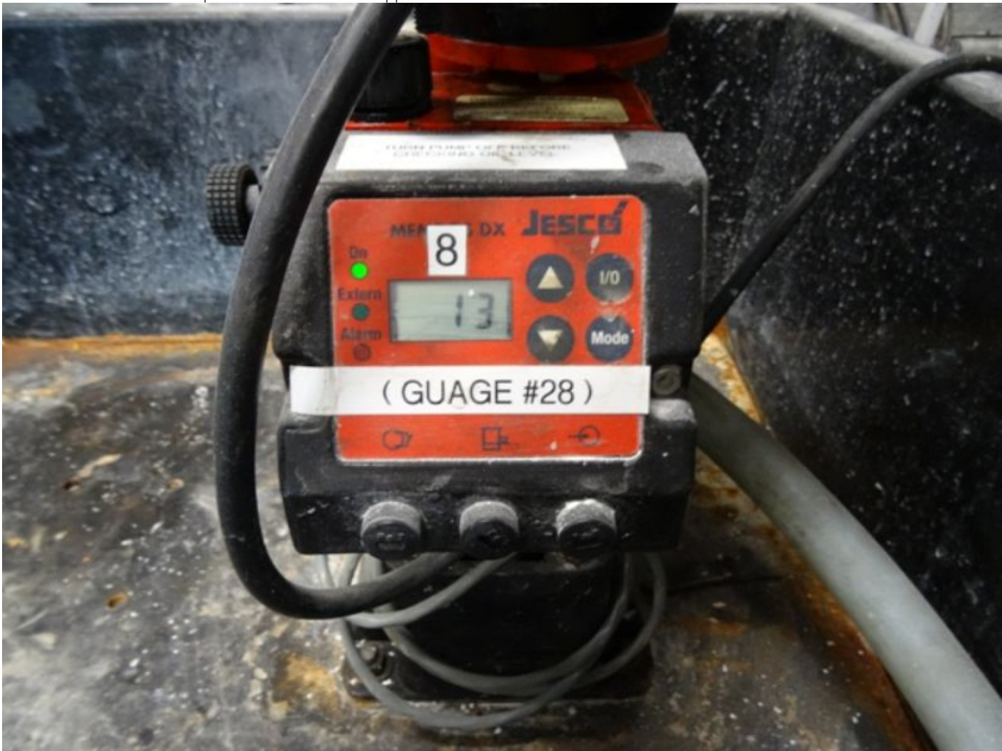
Figure 4 Chlorine pump
