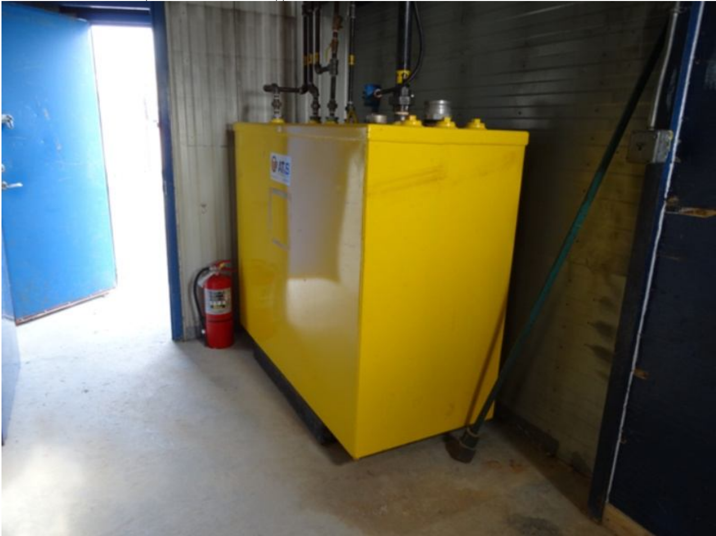
Figure 2 Day tank inside Pump station
