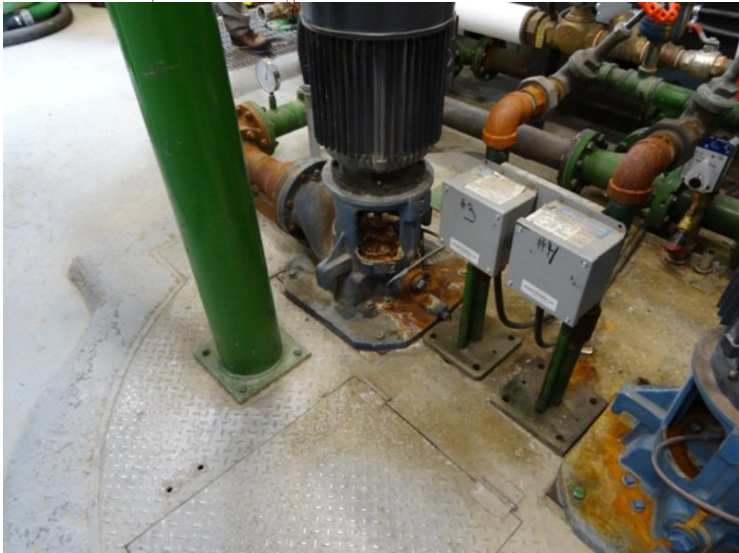
Figure 8 Rusted out pump in service in building
