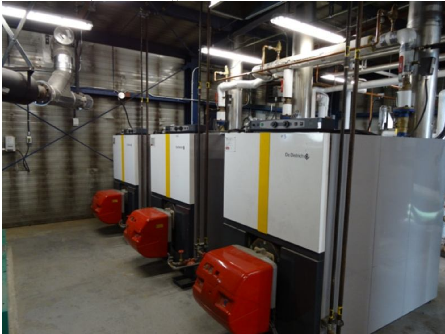
Figure 6 Boilers to heat water to keep both the distribution lines and recirculation lines open
