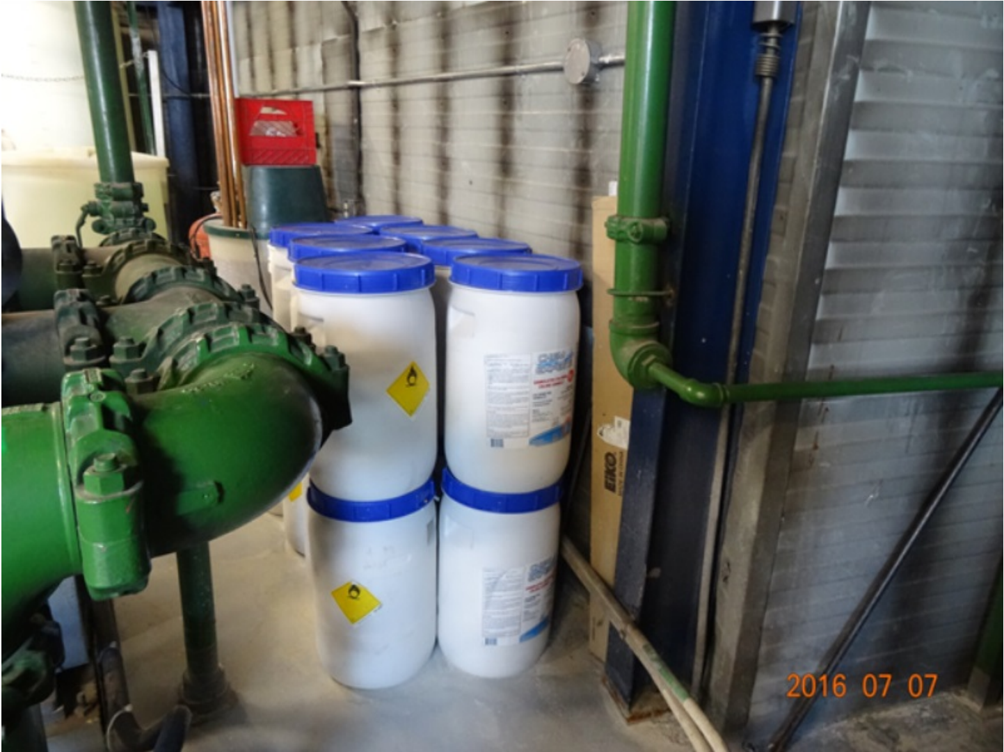
Figure 3 Chlorine/ chemical storage
