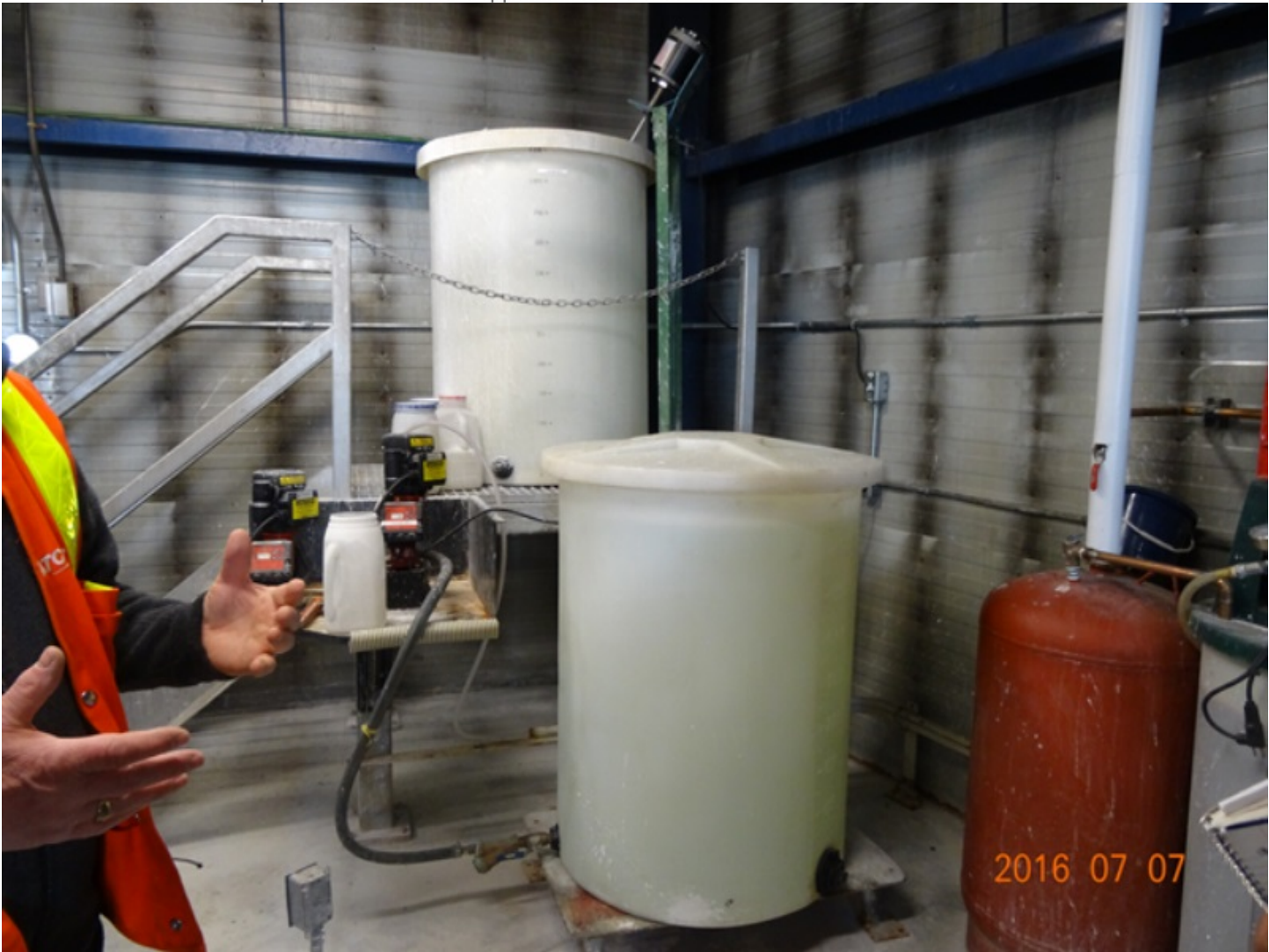
Figure 4 Chlorination system
