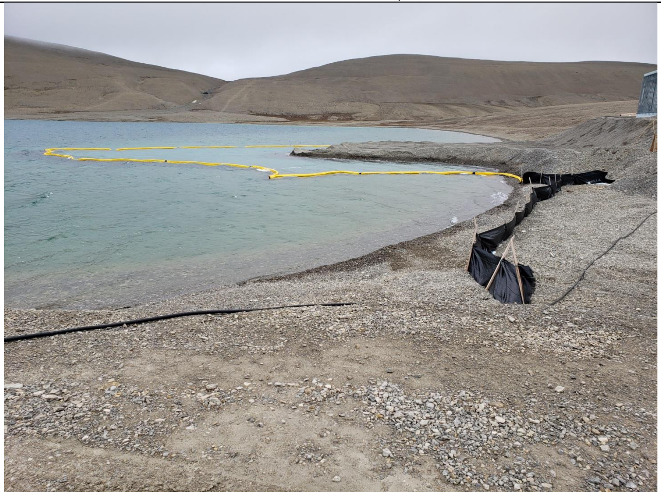
Description: Boom installed in Char lake to mitigate any leaks, or sedimentation.
