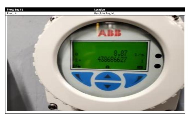
Description: ABB meter observed in the water pump house. 438686627 Litres, 438686.627m<sup>3</sup>
