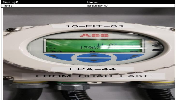
Description: New water meter from Char Lake to Water Treatment Plant – Meter photo skewed by light reflection. Assumed reading at the time of inspection may read 179679814 m³. Photo taken at Water Treatment Plant.
