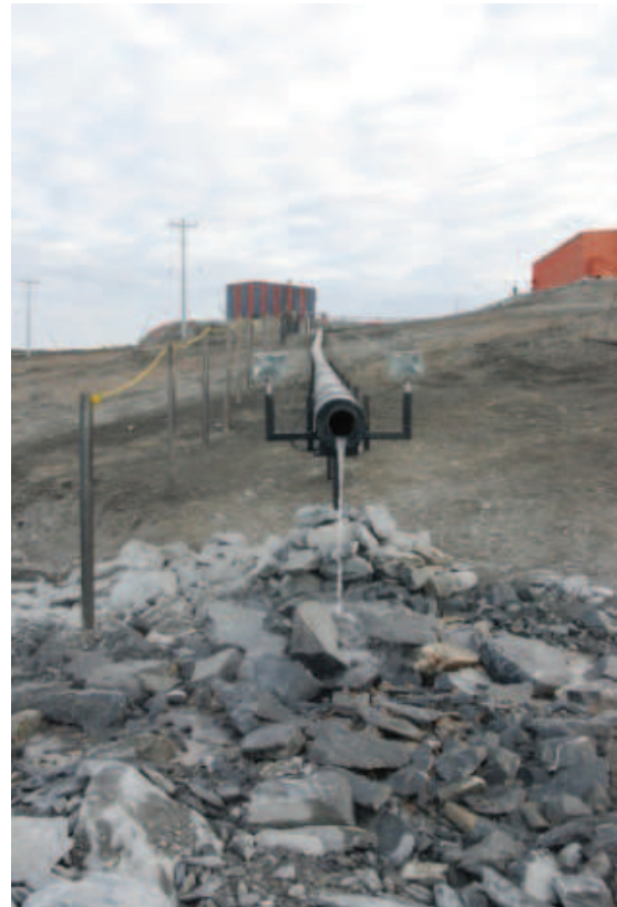
Figure 1.2. The discharge pipe delivering wastewater to the wetland
