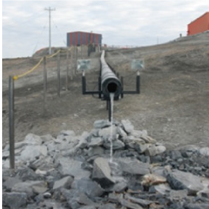
Figure 1-2: The discharge pipe delivering wastewater to the wetland.
