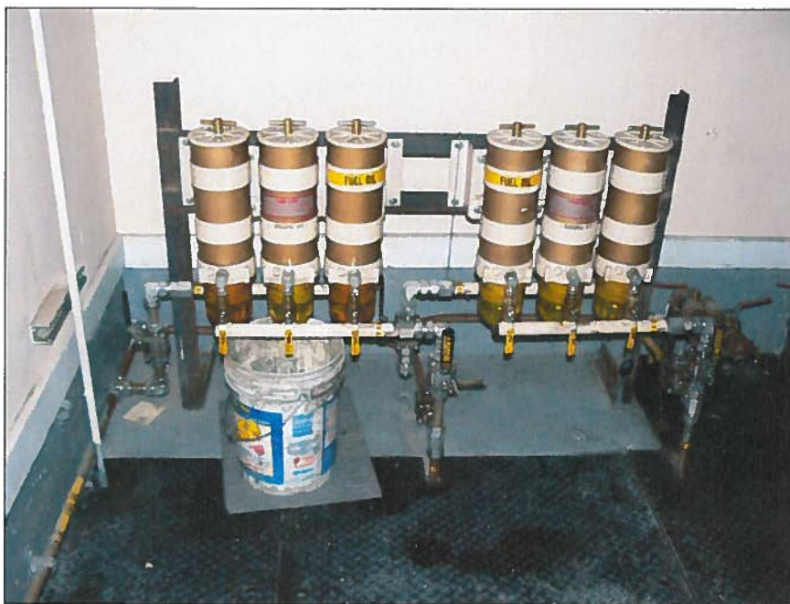
Figure 3 –Fuel Filter Assembly located in the Fuel Room at the Stand-By Power Plant (B-146).
