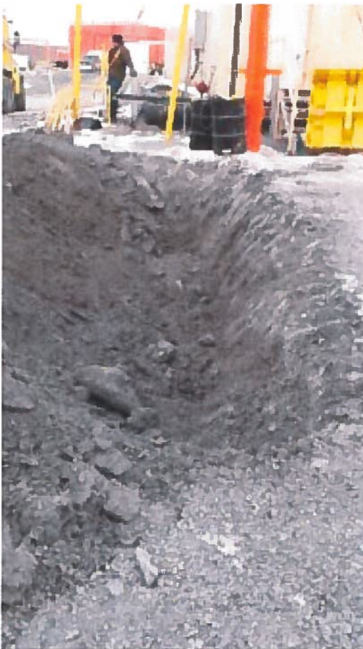
Figure 2 – Excavation of fuel contaminated soils at CFS Alert.
