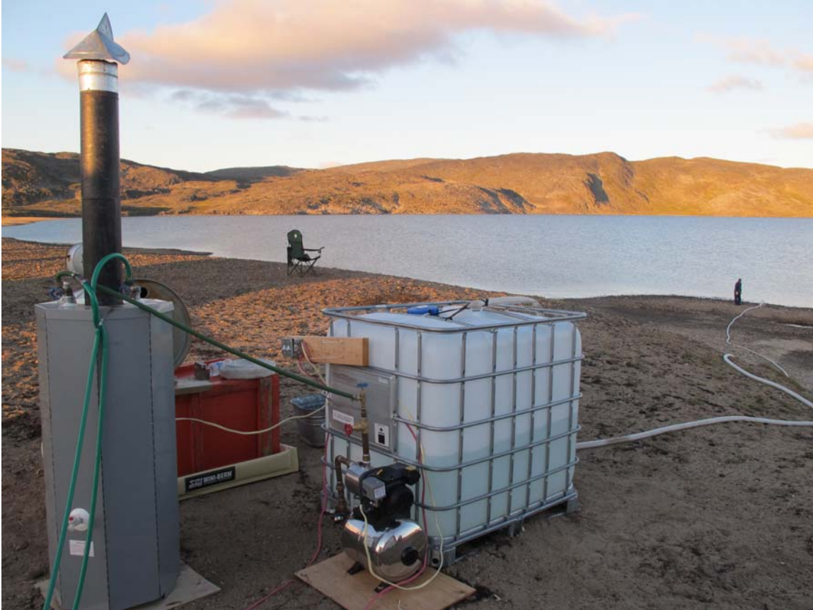
Figure 6: Water pump, container and heater system.
