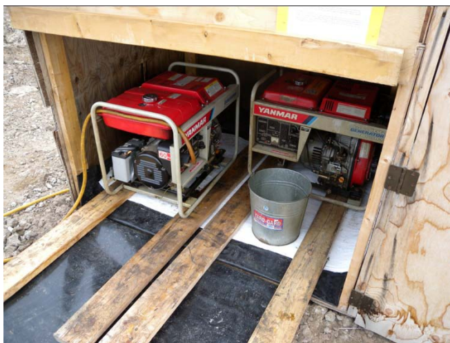
Diagram 9 – Interior of Generator Shed, Showing Diesel Generators & Secondary Containment. (Images Captured in July, 2009)
