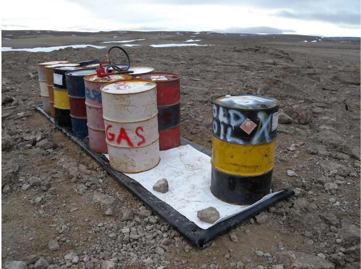
Diagram 3 – Secondary Containment for Permanent Fuel Storage and for Storage of Waste Oil (Image Captured in July, 2009)
