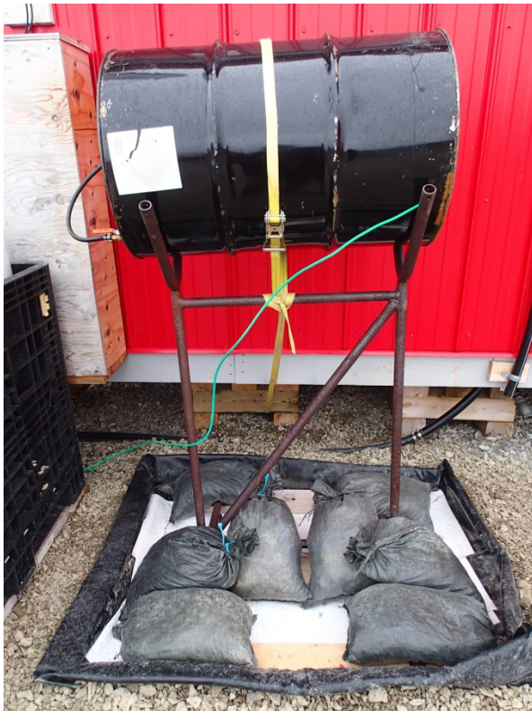
Temporary fuel tank and berm
