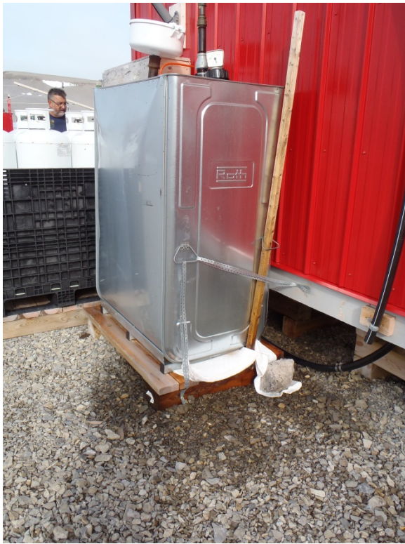
Roth tank showing bowing to outer skin
