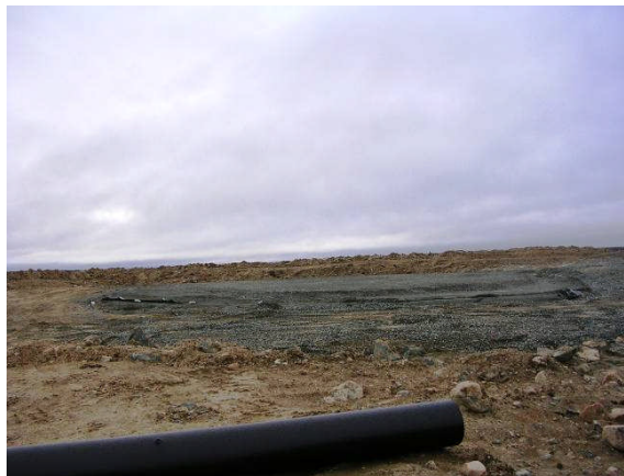
Photo 1: Base and liner of the 5 million litre fuel tank
