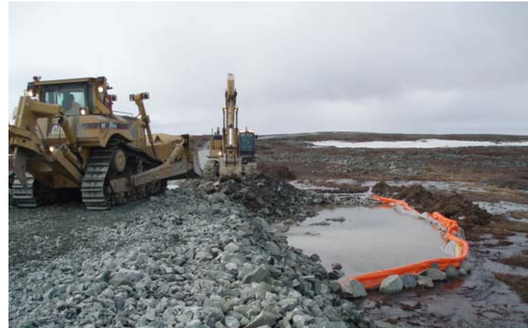
Photo 14. R07 – Sediment settling pond with silt curtain while road is being raised (18Jun07)
