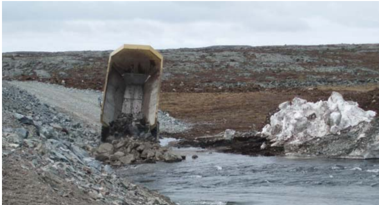
Photo 8. R02 – Adding boulders to stabilize unstable bank area (U/S S side) (17Jun07)
