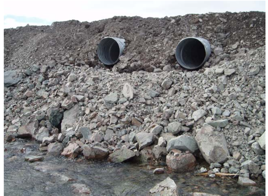
Photo 12. R02 – D/S side showing newly added culverts and road material (19Jun07).
