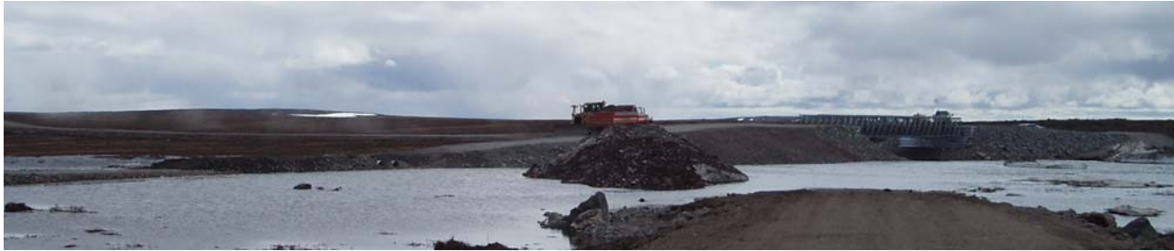
Photo 10. R02 – Road height increase and culvert spillway installation to prevent major instability and erosion on N approach (19Jun07).
