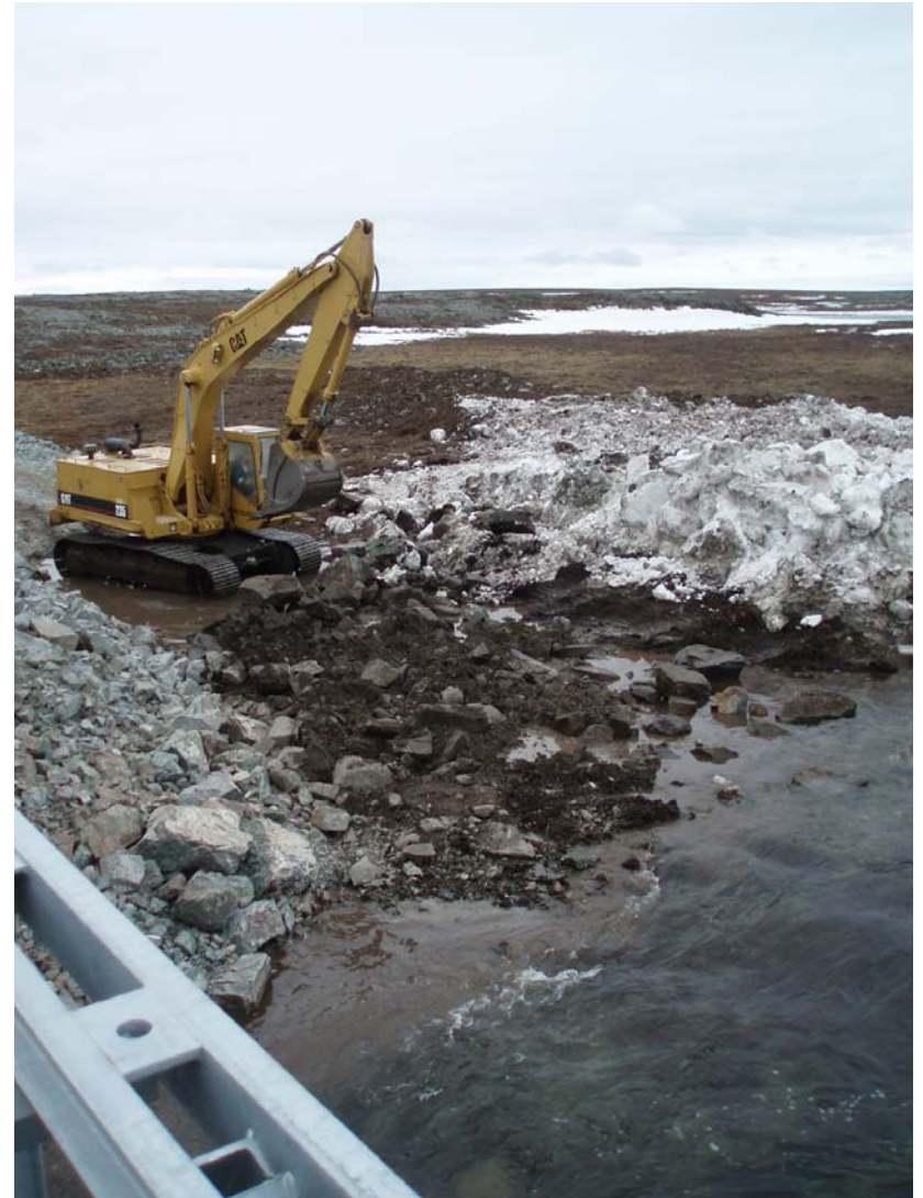
Photo 9. R02 – Adding boulders to stabilize unstable bank area (U/S S side) (17Jun07)
