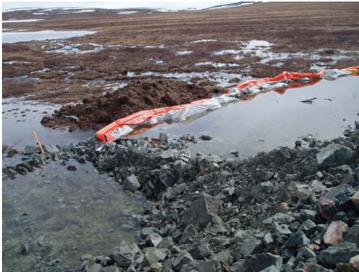
Photo 15. R07 – Settling pond showing clear water (19Jun07)
