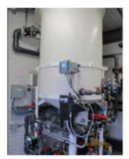
Figure 5-2: Contact Tank Used in NWT Membrane Plants
