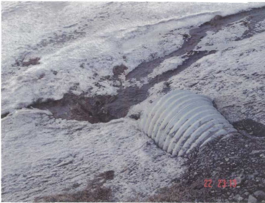
Photo 5. Culvert that drains Lagoon effluent to Arctic Bay.
