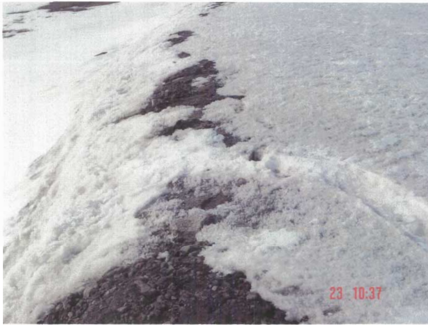
Photo 13. Breach in New Sewage Lagoon berm.
