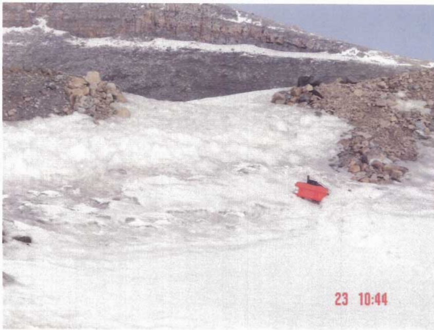
Photo 15. Location of New Sewage Lagoon berm breach.
