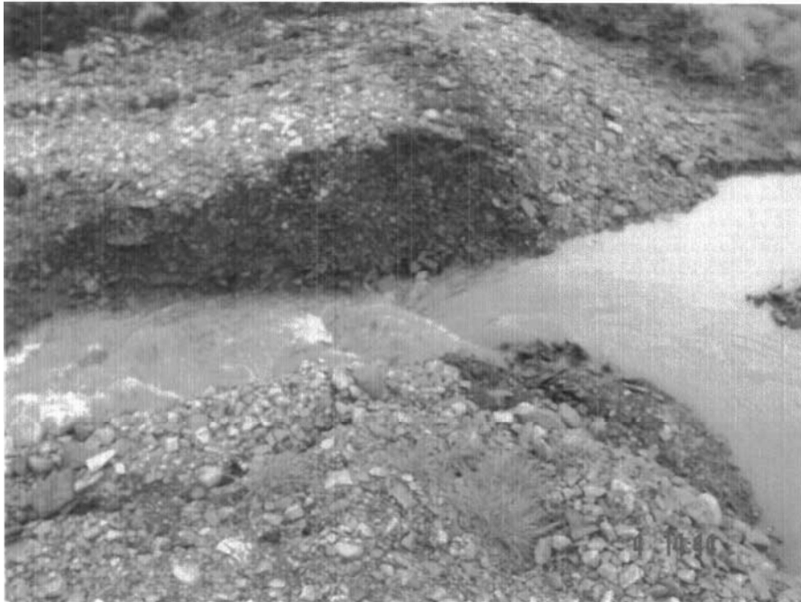
Photo 27. Shale and coarse aggregate material shown in wetlands dispersion berm. Excessive flow in spillway.
