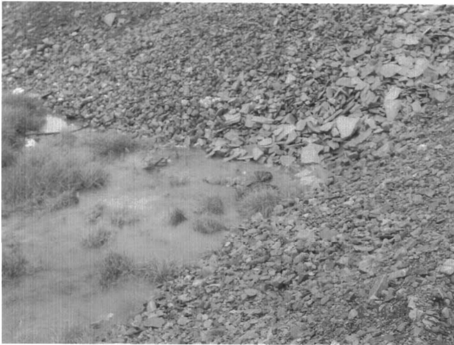
Photo 19. Excessive seepage at (Old-summer Sewage Lagoon).
