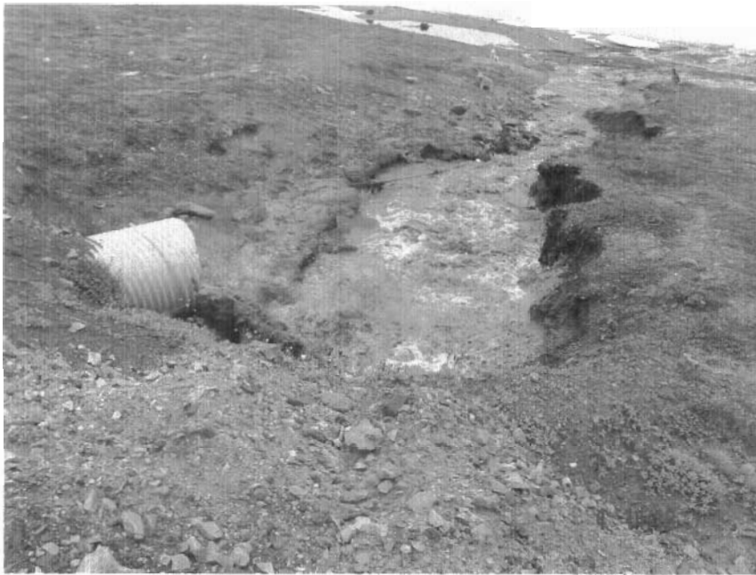
Photo 13. Erosion on discharge side of Arctic Bay Road, Erosion caused by runoff and sewage effluent.
