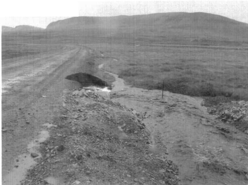
Photo 12. Erosion to Arctic Bay road caused by Runoff and sewage effluent. Sewage sample N 73.0153.6 W 85.0511.5.
