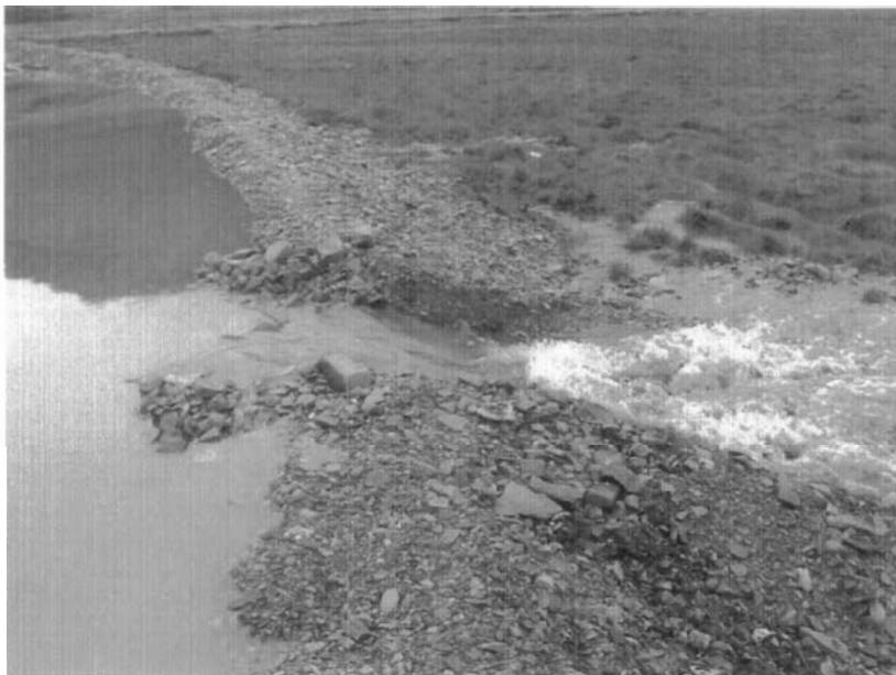
Photo # 16. Excessive sewage effluent shown at berm #2 spillway.
