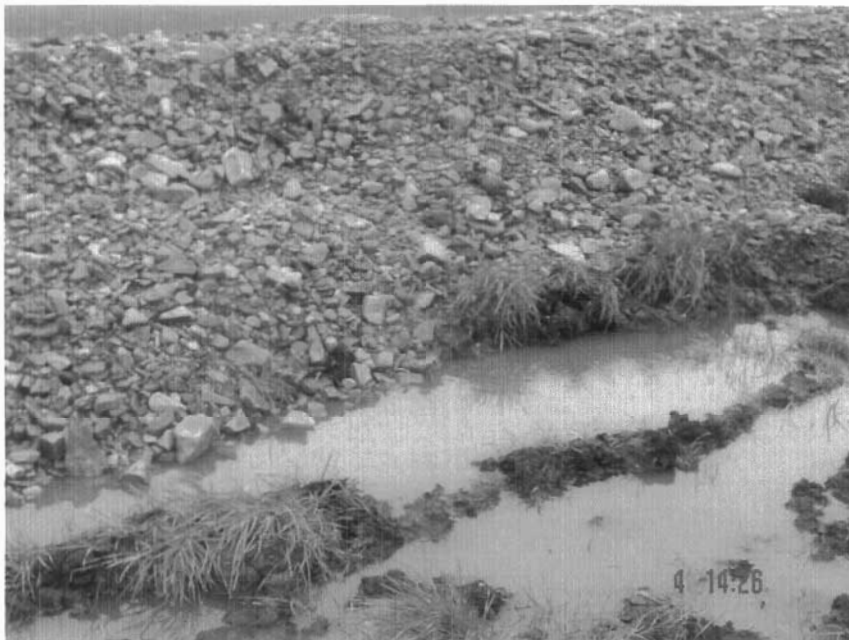
Photo 13. Erosion on discharge side of Arctic Bay Road, Erosion caused by runoff and sewage effluent.
