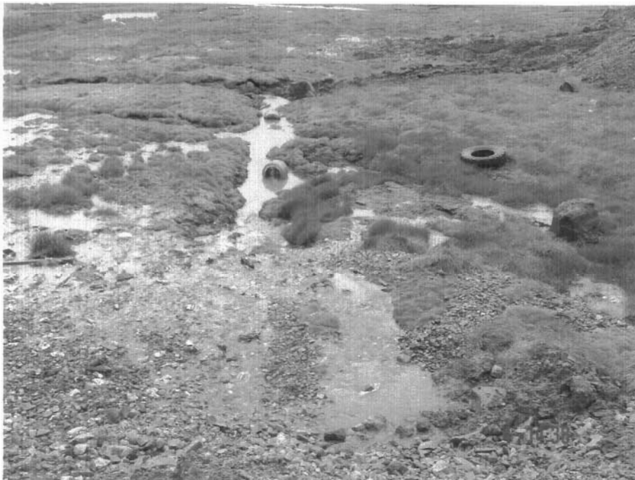
Photo 19. Excessive seepage at (Old-summer Sewage Lagoon).
