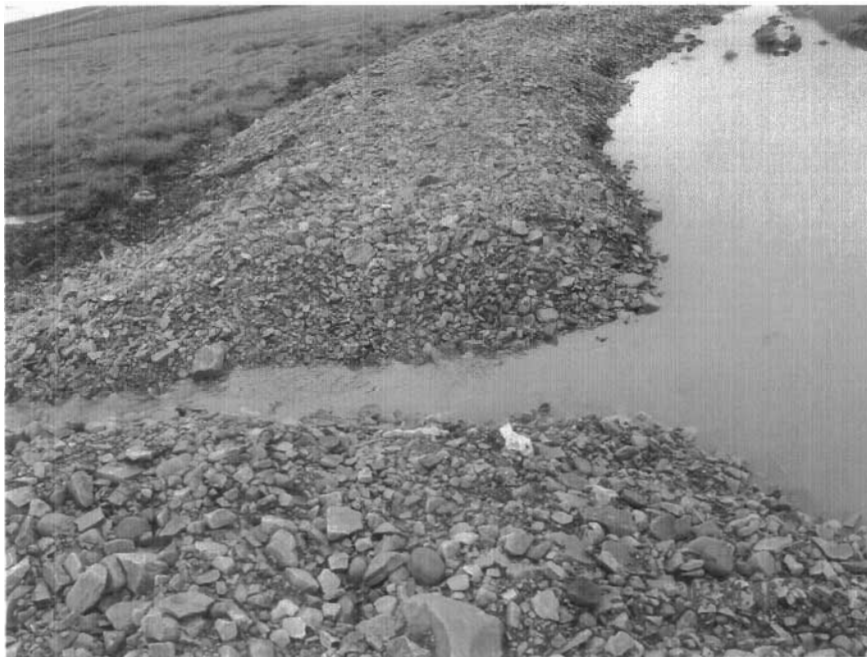
Photo 28. Spillway shown in berm #2, shown operating due to improper material in berm.
