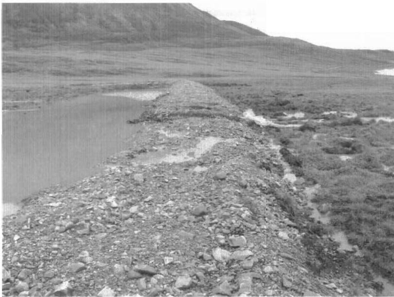
Photo 29. Seepage shown circumventing dispersion berm # 1.
