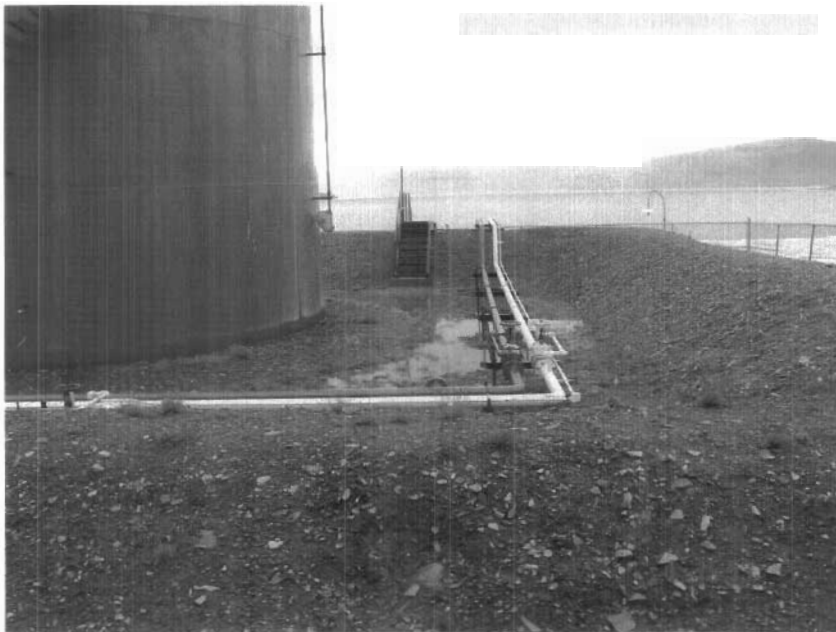
Photo 36. Tank Farm berm in good condition with minimal contained water.
