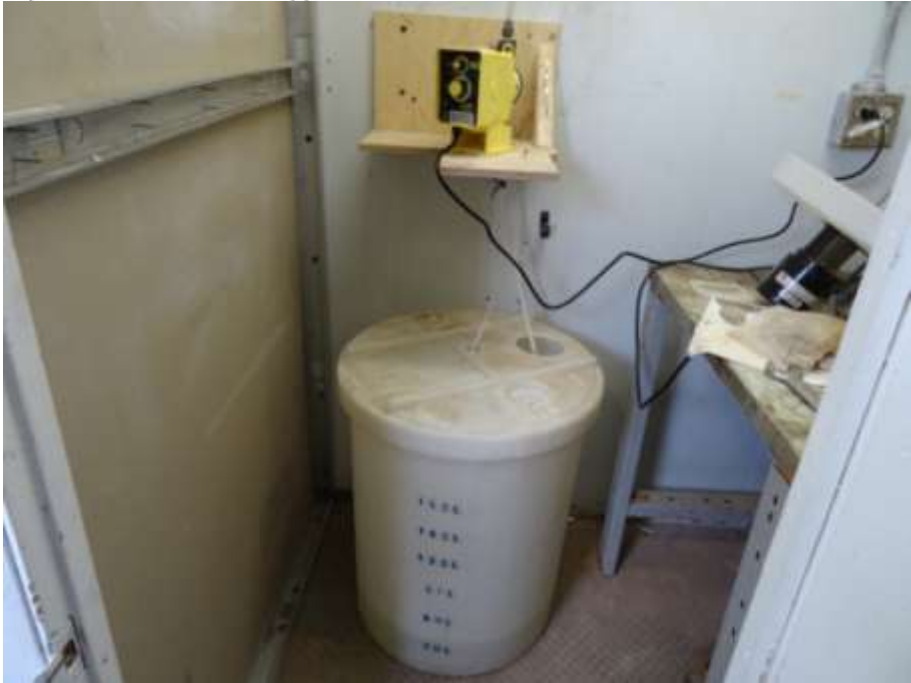
Figure 4 Chlorination system- Tank low (No mixing Tank)
