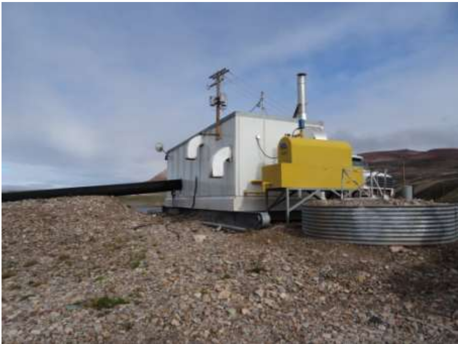
Figure 2 Intake- Double walled back up fuel tank
