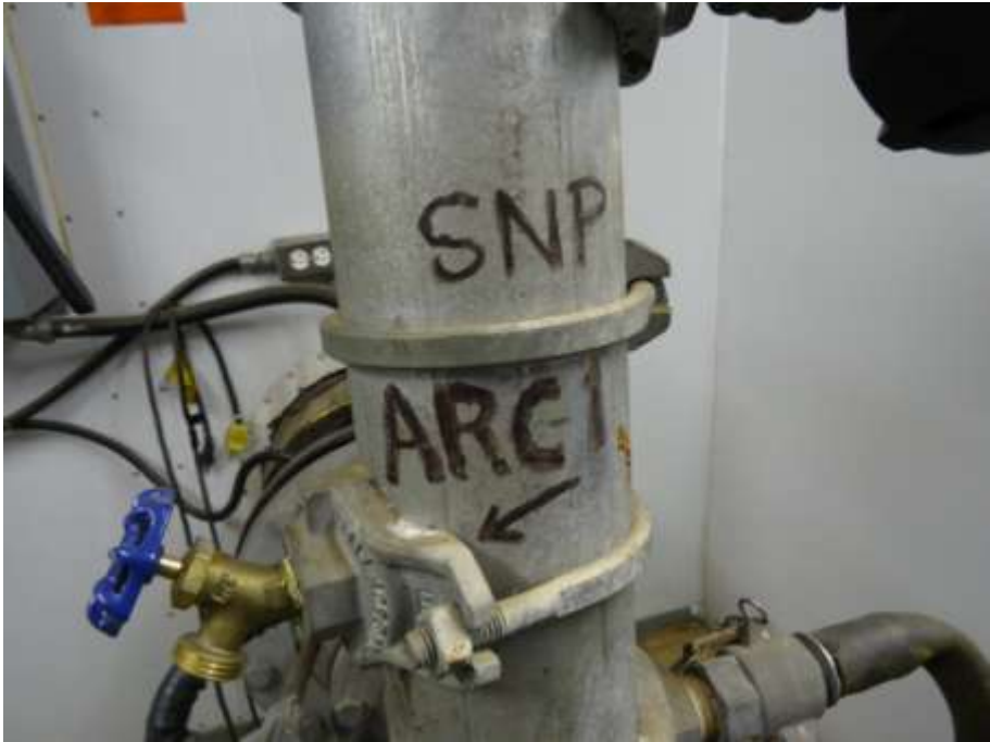
Figure 5 Raw water sampling port in the In-take station
