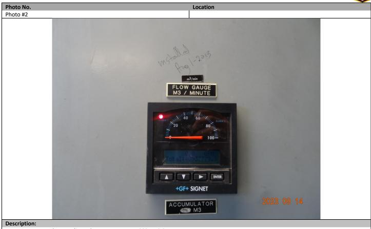
Water treatment plant totalizer. Flow gauge meter: 40937779.0
