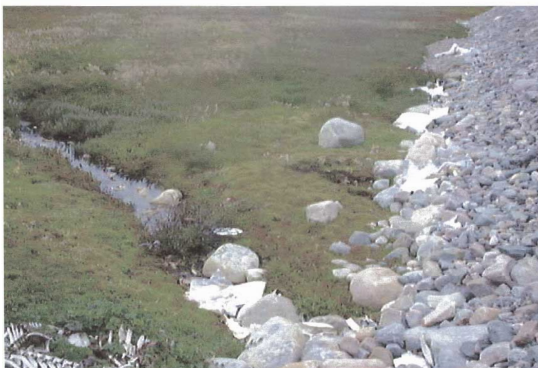
figure 8. Pooled water at the toe of the solid waste disposal facility; 2000/08/29.
