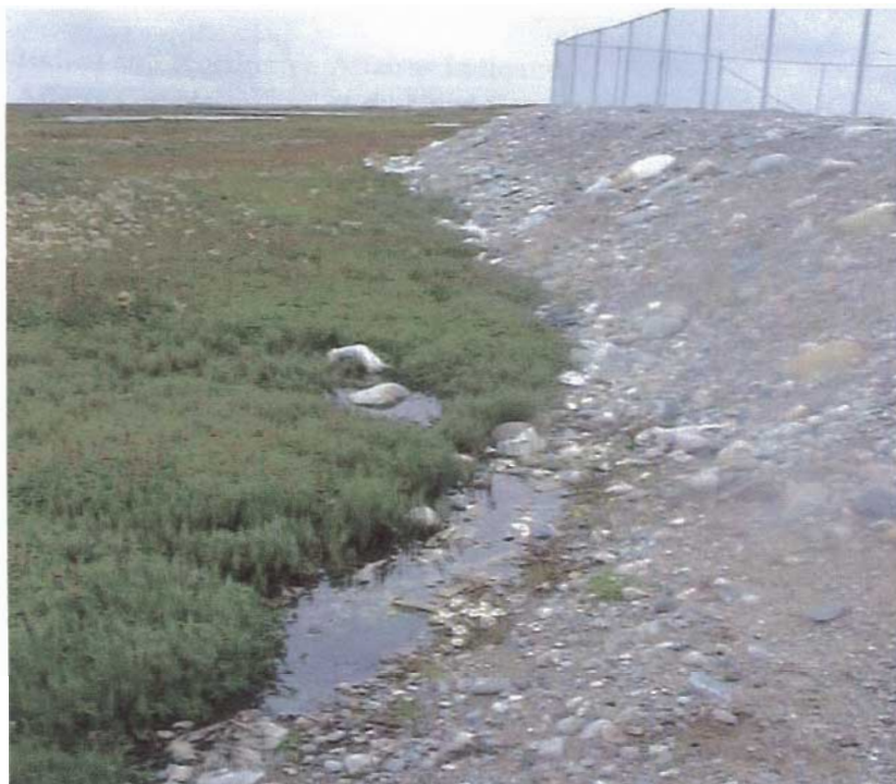
figure 7. Pooled water at the toe of the solid waste disposal facility; 2000/08/29.
