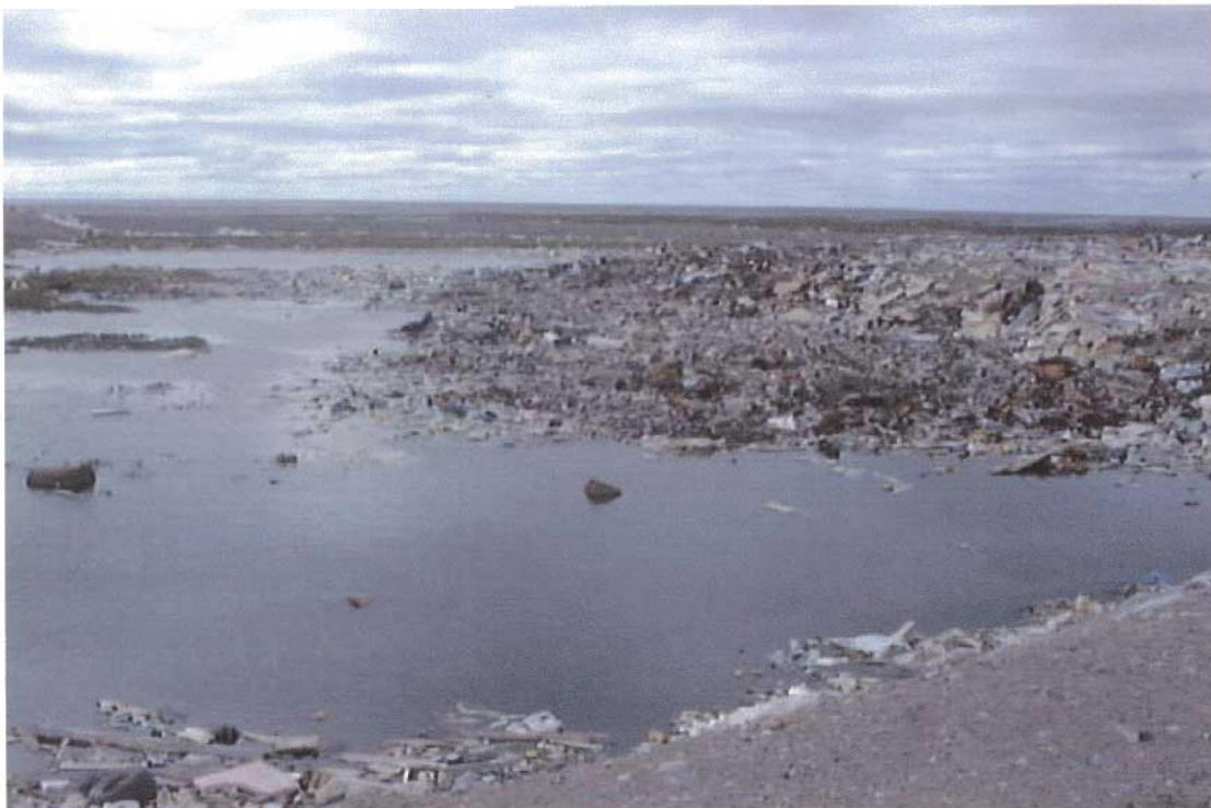
figure 5. Pooled water along the toe of the solid waste disposal facility; 2001/08/30.
