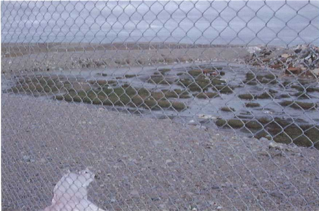
figure 7. Pooled water along the toe of the solid waste disposal facility; 2001/08/30.
